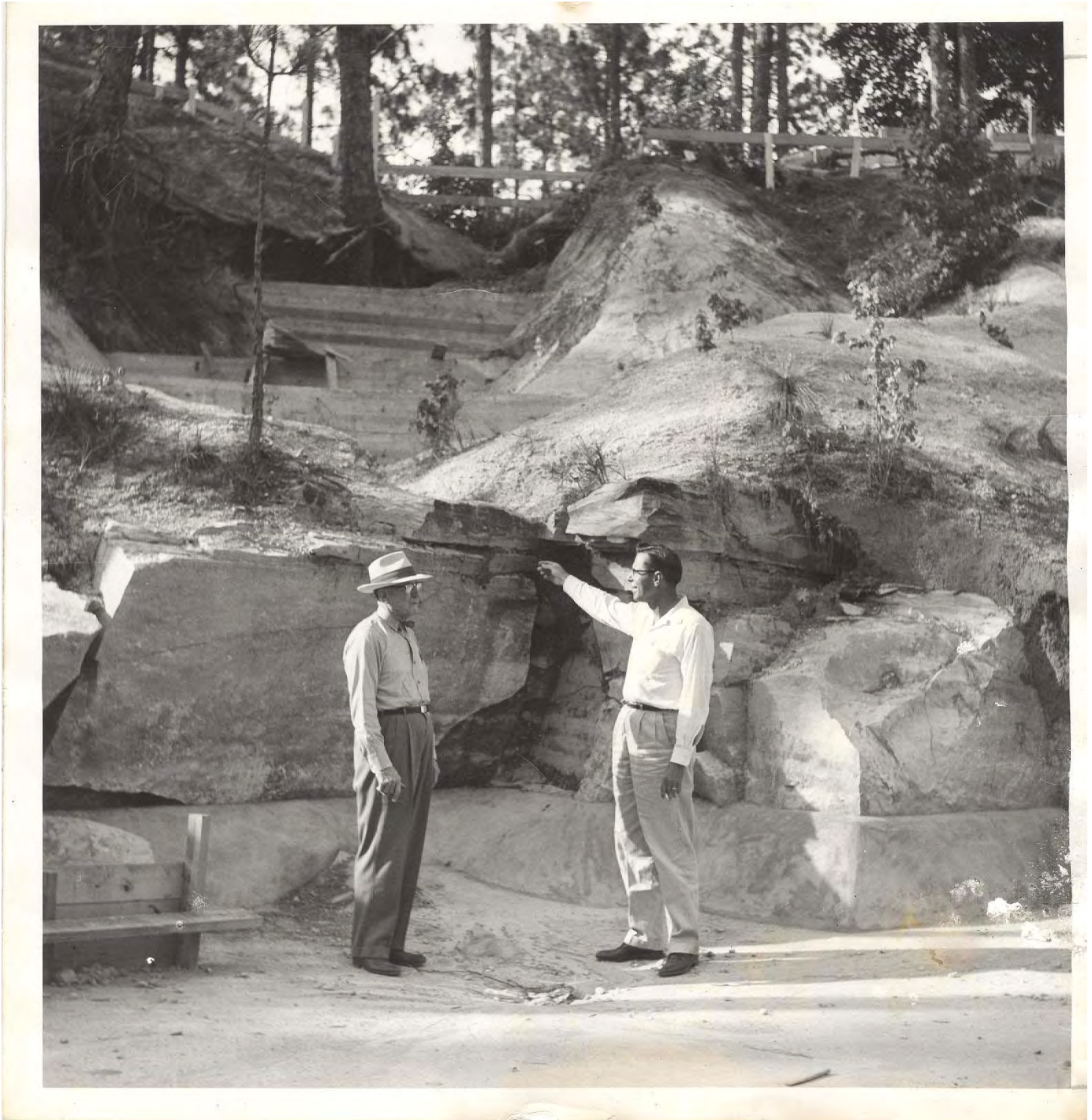
Figure 4. A.J. Hodges and a worker discussing plans during the gardens' construction (notice the original quarry in the background). Image courtesy of the Hodges Gardens Archives.
