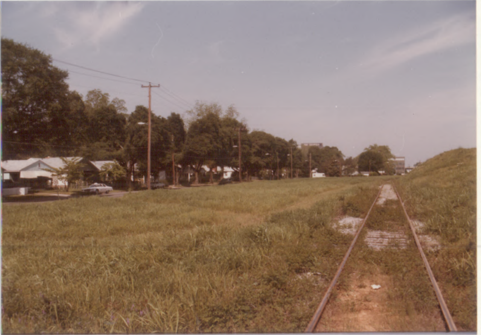
15. Railroad tracks along levee at Second Street looking northwest
