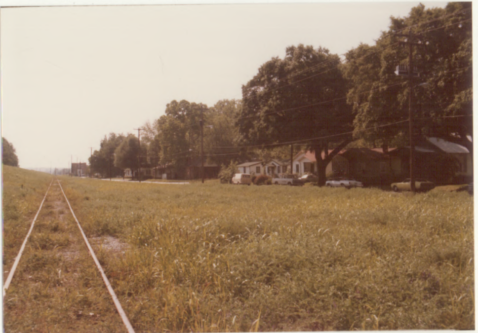
16. Railroad tracks along levee at Second Street looking southeast
