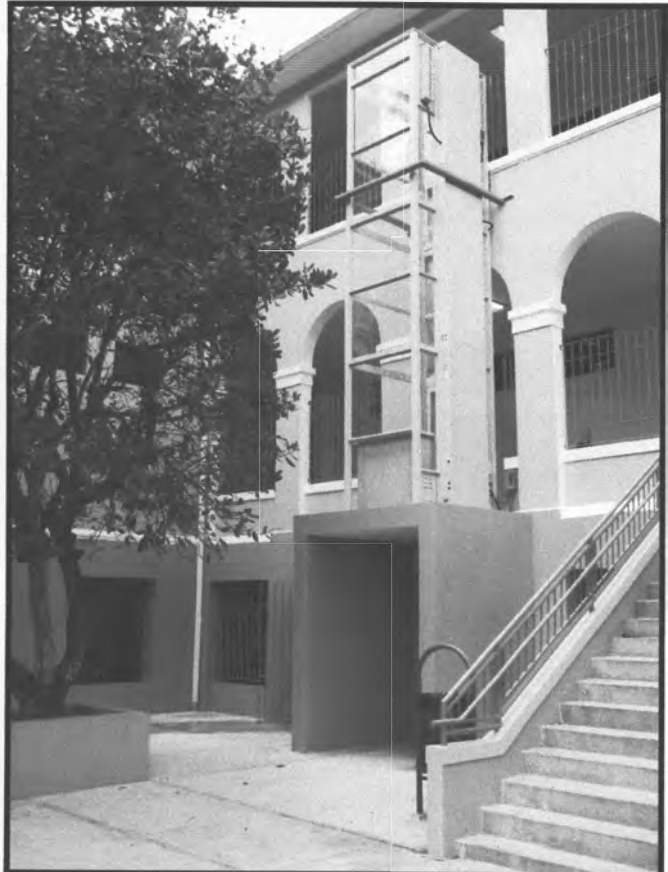
Figure 15. Close up of the traction elevator built in the northern façade. Photo taken on 09/20/12.
