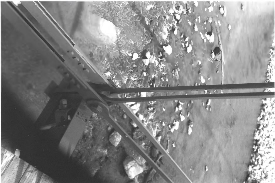
Walnut Street Bridge Wakasha Co., Mn 014396-16
