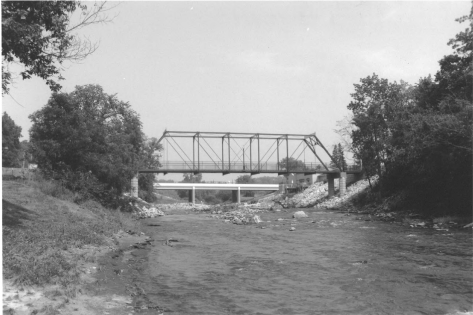
Walnut Street Bridge Wabasha Co., Minn 014396-11
