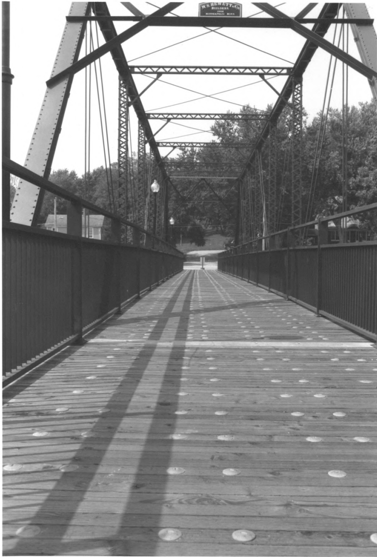
Walnut Street Bridge Wabasha Co., MN 014396-21
