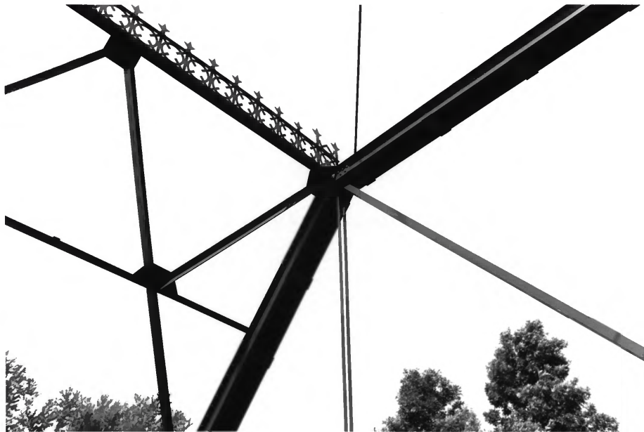
Walnut Street Bridge Wabasha Co., MN 014396-19
