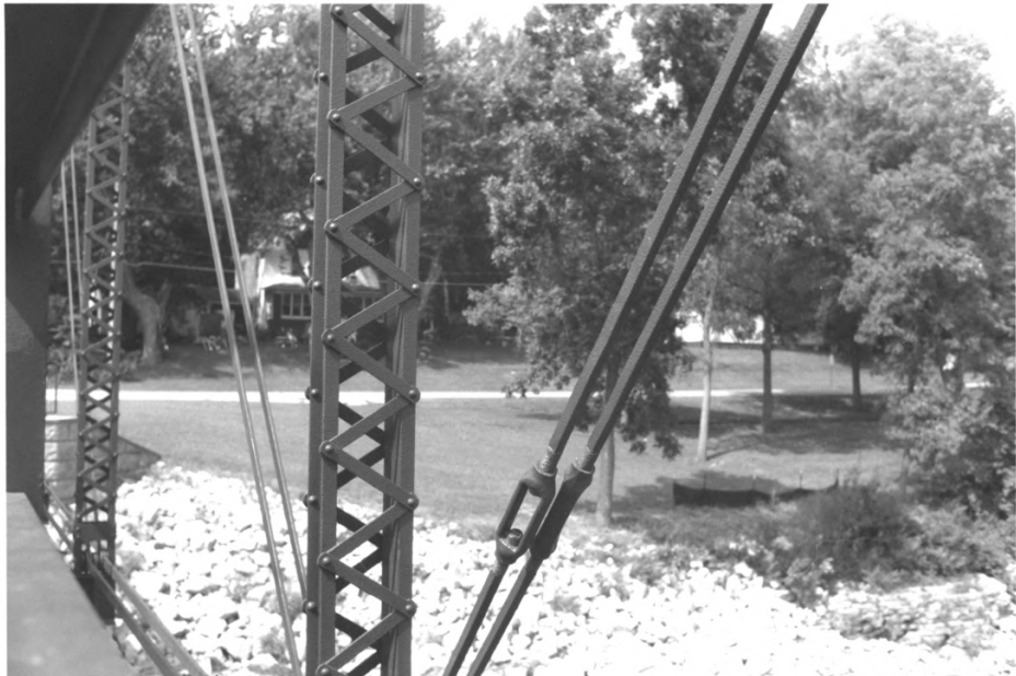
Walnut Street Bridge Wakasha Co., Mn 014396-20
