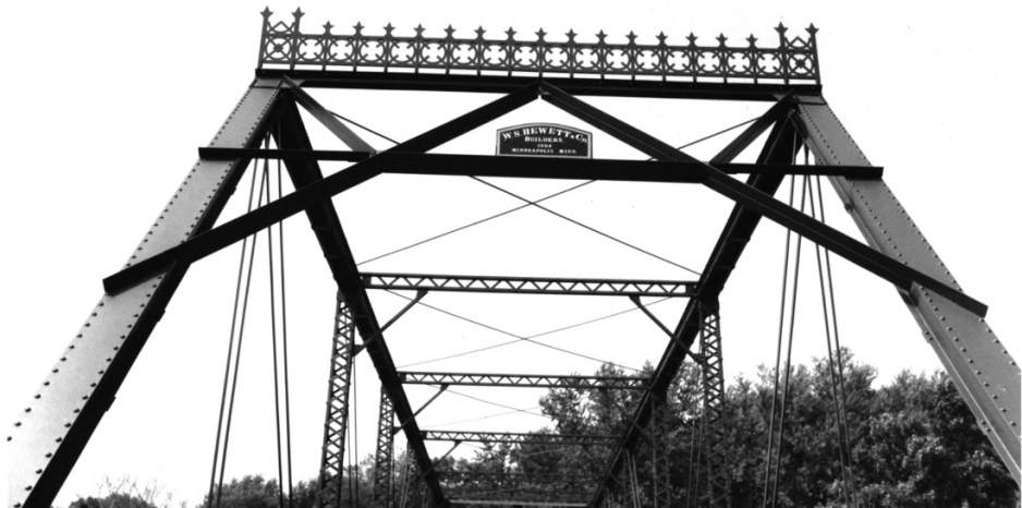
Walnut Street Bridge Wabasha Co., Mn 014396-8
