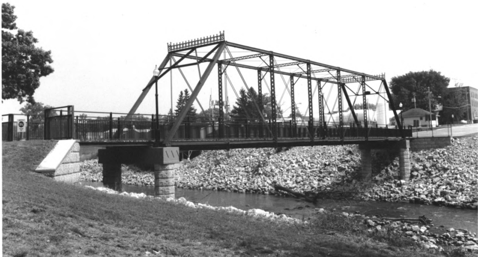
Walnut Street Bridge Wabasha Co., Mn 014396-9
