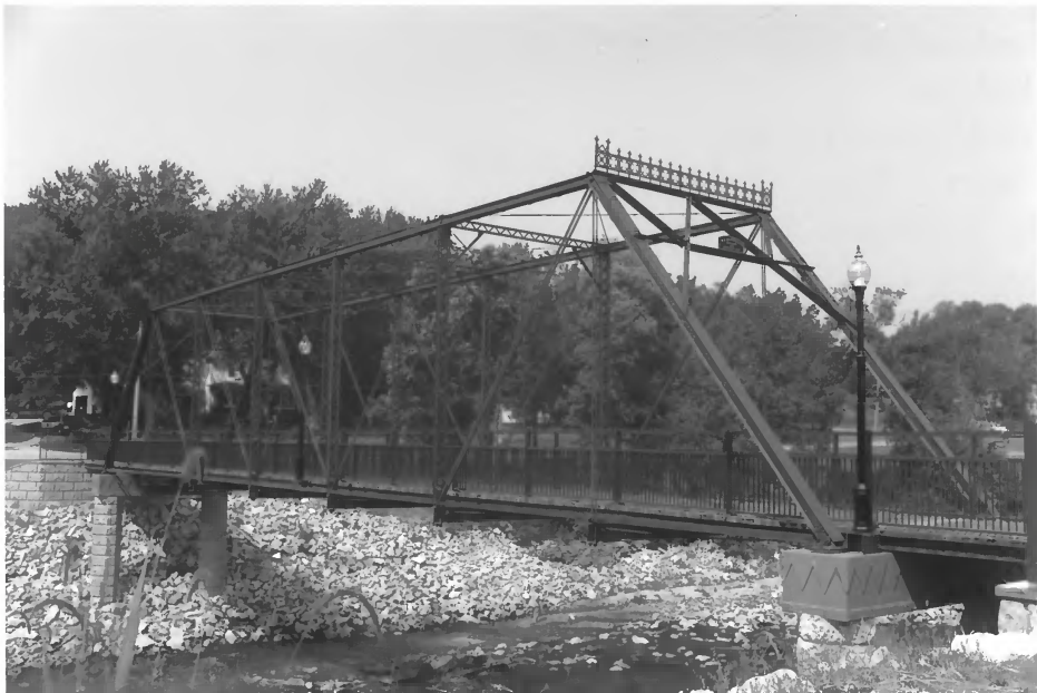
Walnut Street Bridge Wabasha Co., Mn 014396-3
