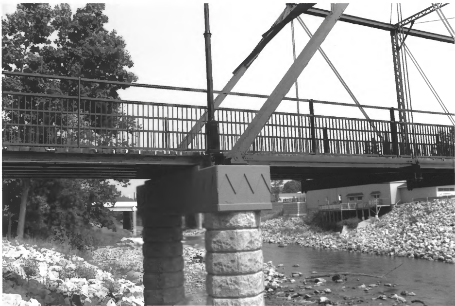
Walnut Street Bridge Wabasha Co., Mn 014396-14
