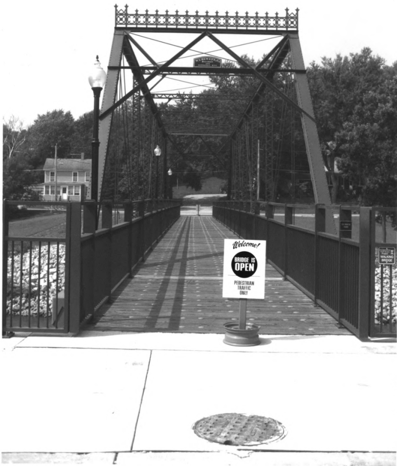
Walnut Street Bridge Wabasha Co., MN 014396-6
