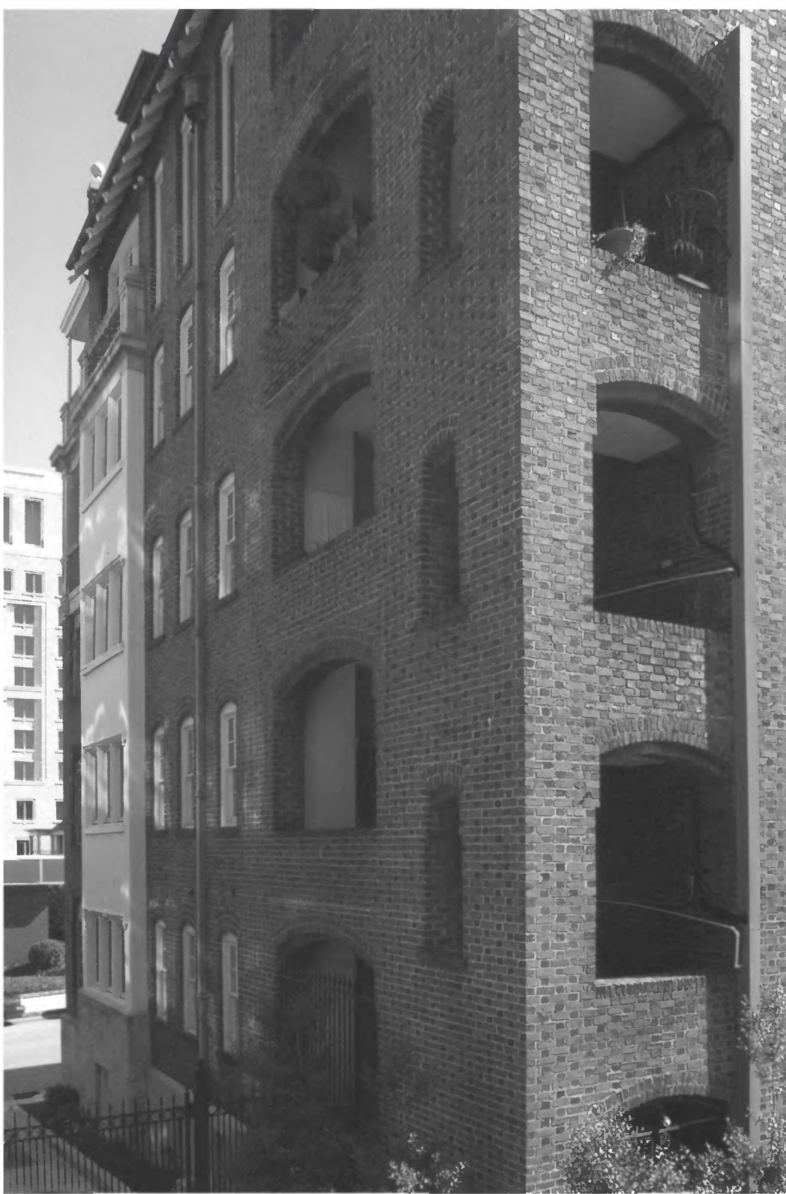
Palmer House and Phelan House Apartments Fulton County, Georgia Photograph 4 of 25
