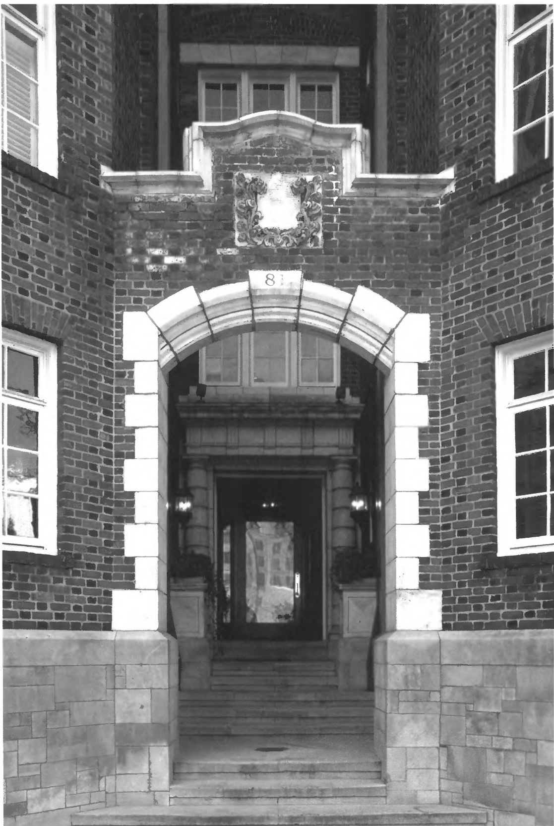
Palmer House and Phelan House Apartments Fulton County, Georgia Photograph 2 of 25
