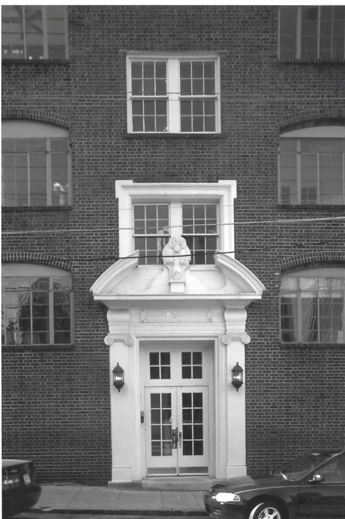
Palmer House and Phelan House Apartments Fulton County, Georgia Photograph 19 of 25
