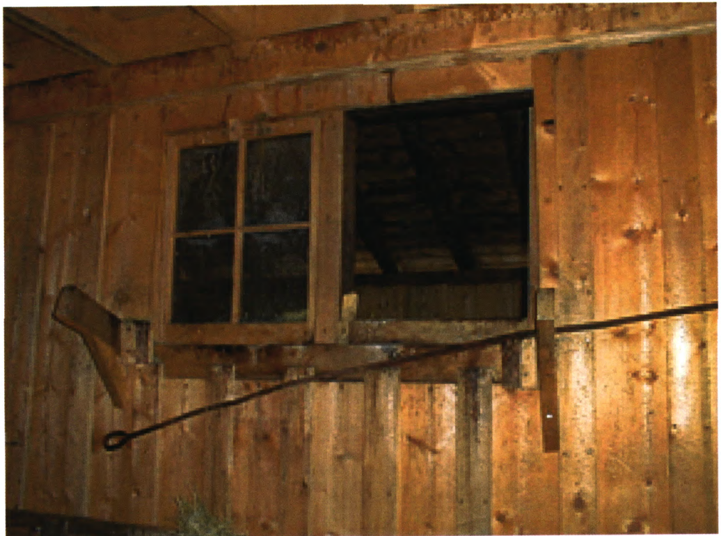
Interior wall – East room – existing conditions
