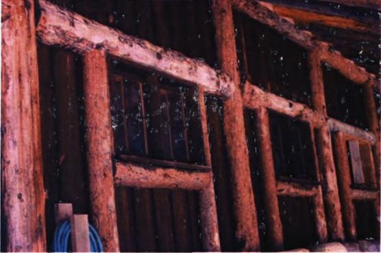
Restored windows, September 2003, photo by Isabel Erickson
