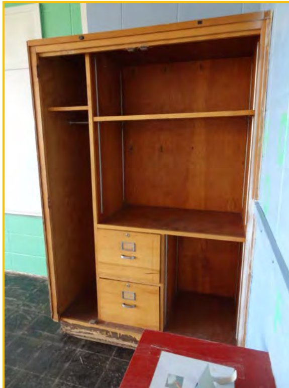
Figure 36. Original cabinetry in elementary building. Photographed by the author, December 15-16, 2017.
