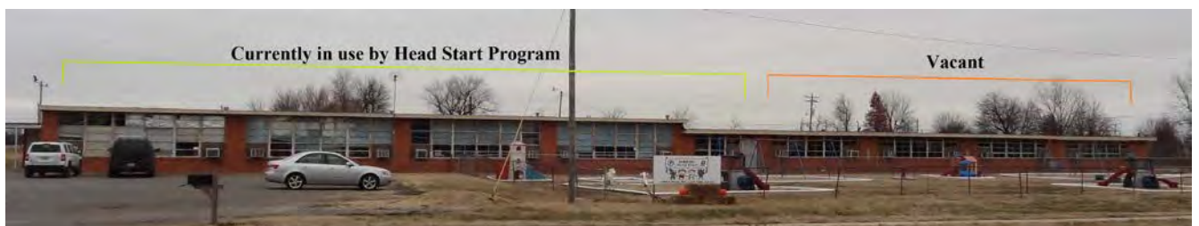
Figure 23. Showing south elevation of elementary building, c. 1961, with current use labeled. Facing north. Photographed by the author, December 15-16, 2016.
