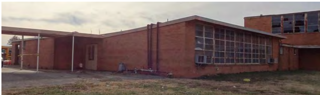
Figure 14. East elevation of the high school building, camera looking southeast. Photographed by the author, December 15-16, 2016.
