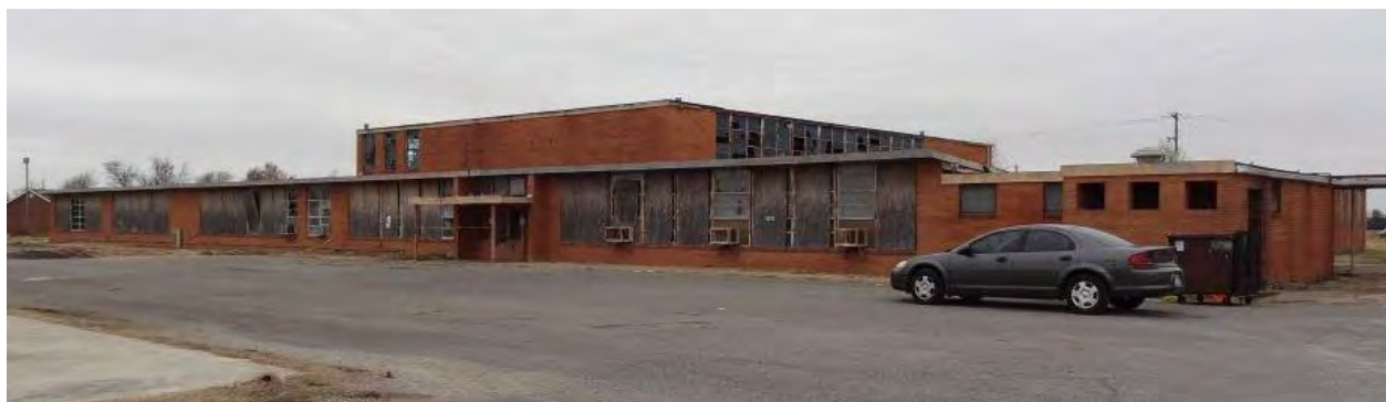
Figure 8. High school building. Camera facing west. Photographed by the author, December 15-16, 2016.
