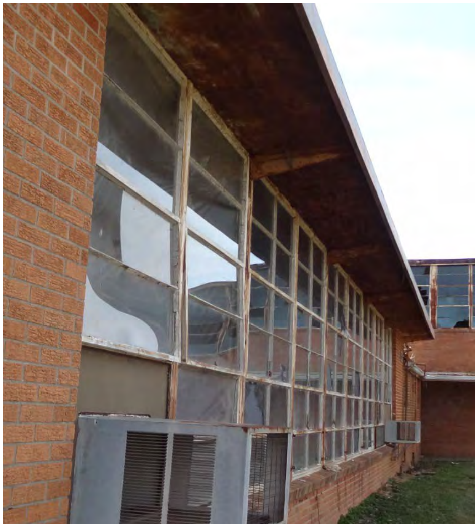
Figure 10. Photo illustrating expanse of windows with functioning awning windows and fixed panes. Rear of high school, camera facing southwest. Photographed by the author, December 15-16, 2016.
