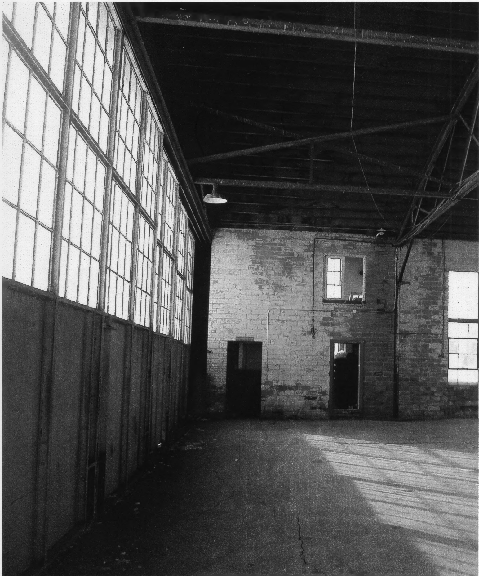
HASTINGS MUNICIPAL AIRPORT HANGAR - Building No. 1 ADAMS COUNTY, NE SUPPLEMENTAL PHOTO 10/3
