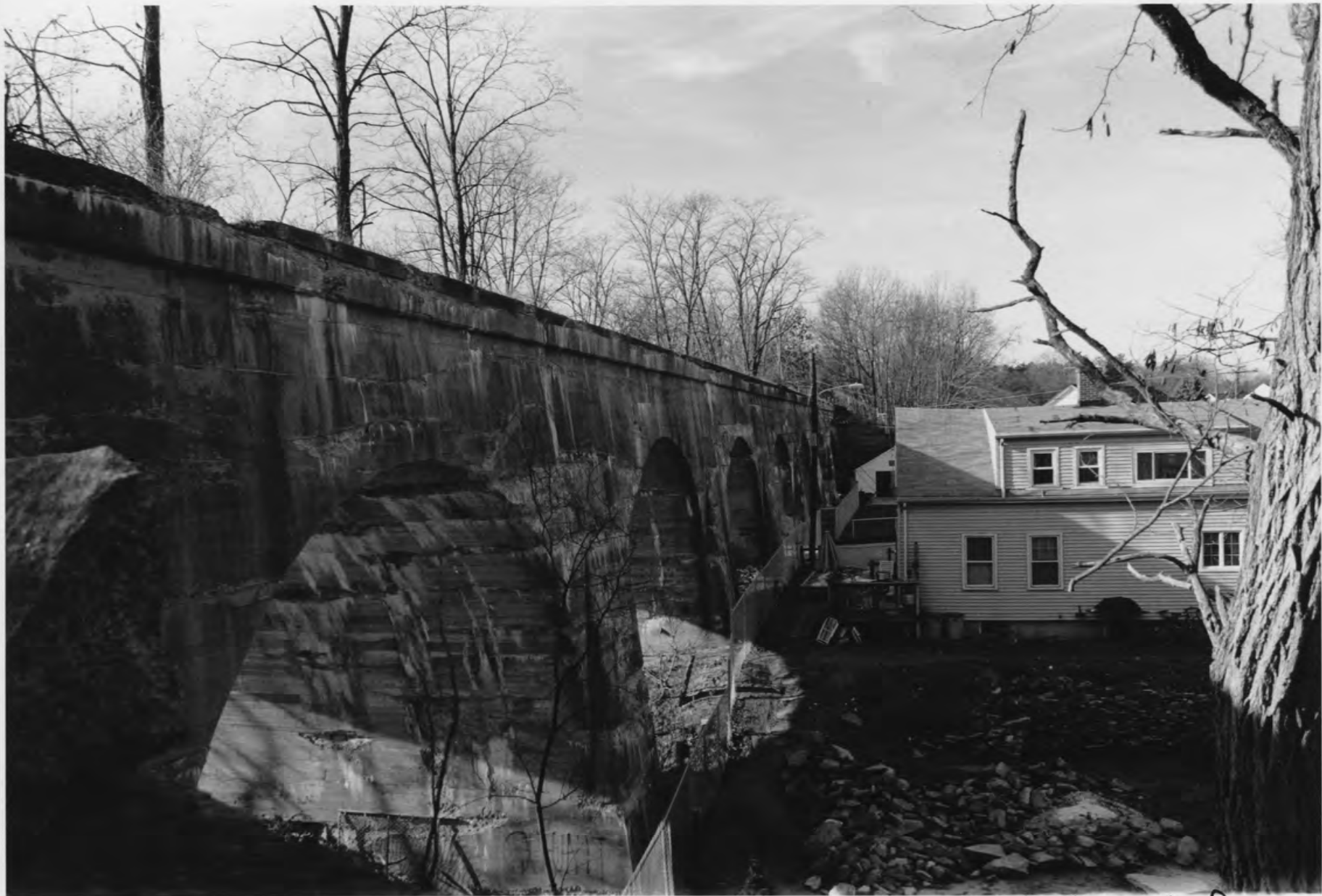
Blackstone Viaduct Blackstone, MA No. 2
