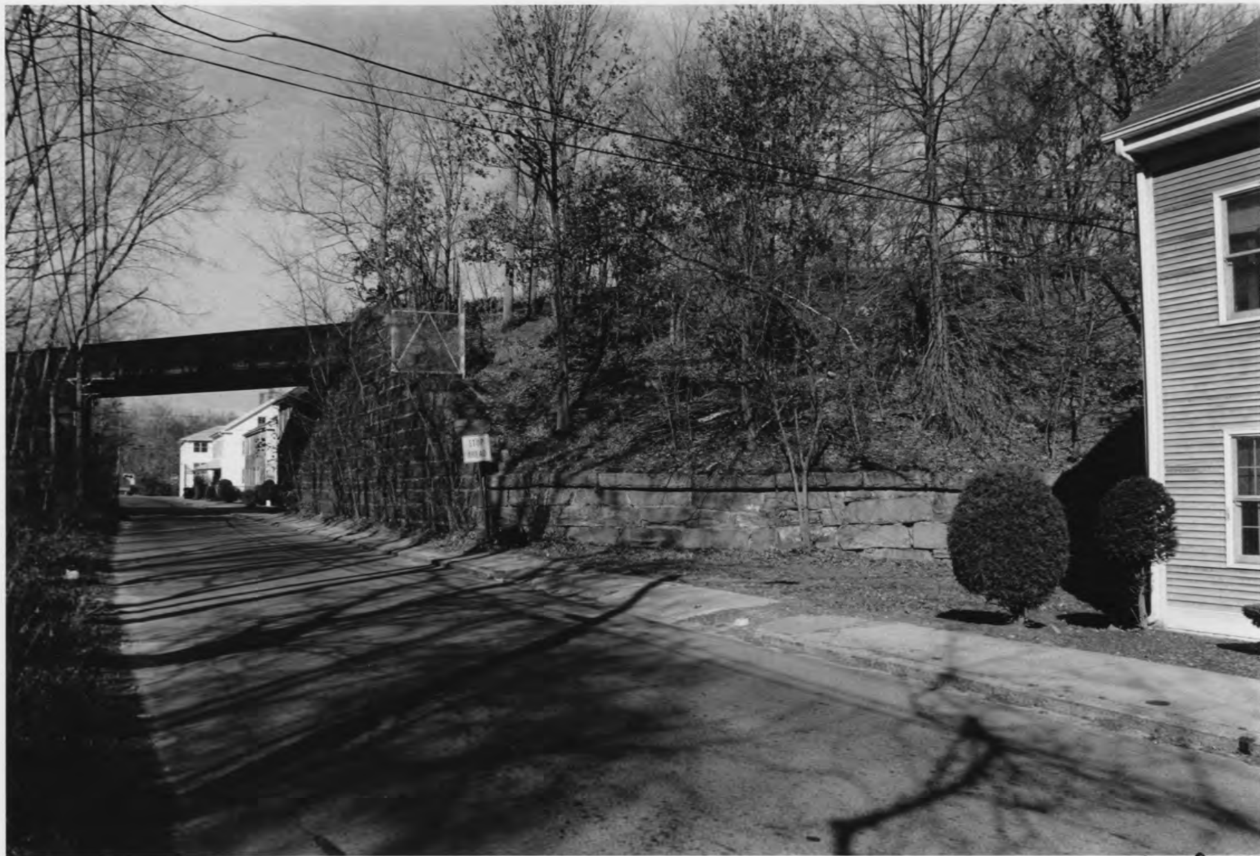
Blackstone Viaduct Blackstone, MA No. 5
