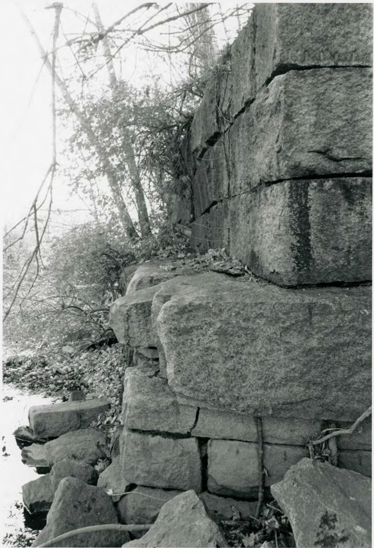
Blackstone Viaduct, Blackstone, MA No. 3
