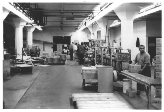
2. Sacramento, California 3. Brian Halloway 4. March, 1980 5. 711 J Street, Sacramento, California 6. General overview of a typical warehouse construction showing mushroom headed reinforced column and beam system. Photo view is south. 7. Photo No. 17. of 21
