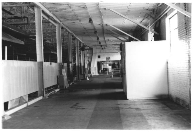
4. March, 1980 5. 711 J Street, Sacramento, California 6. General view of side area of main building showing steel post and beam support system and wood frame roof system. Photo direction is north. 7. Photo No. 16. of 21
