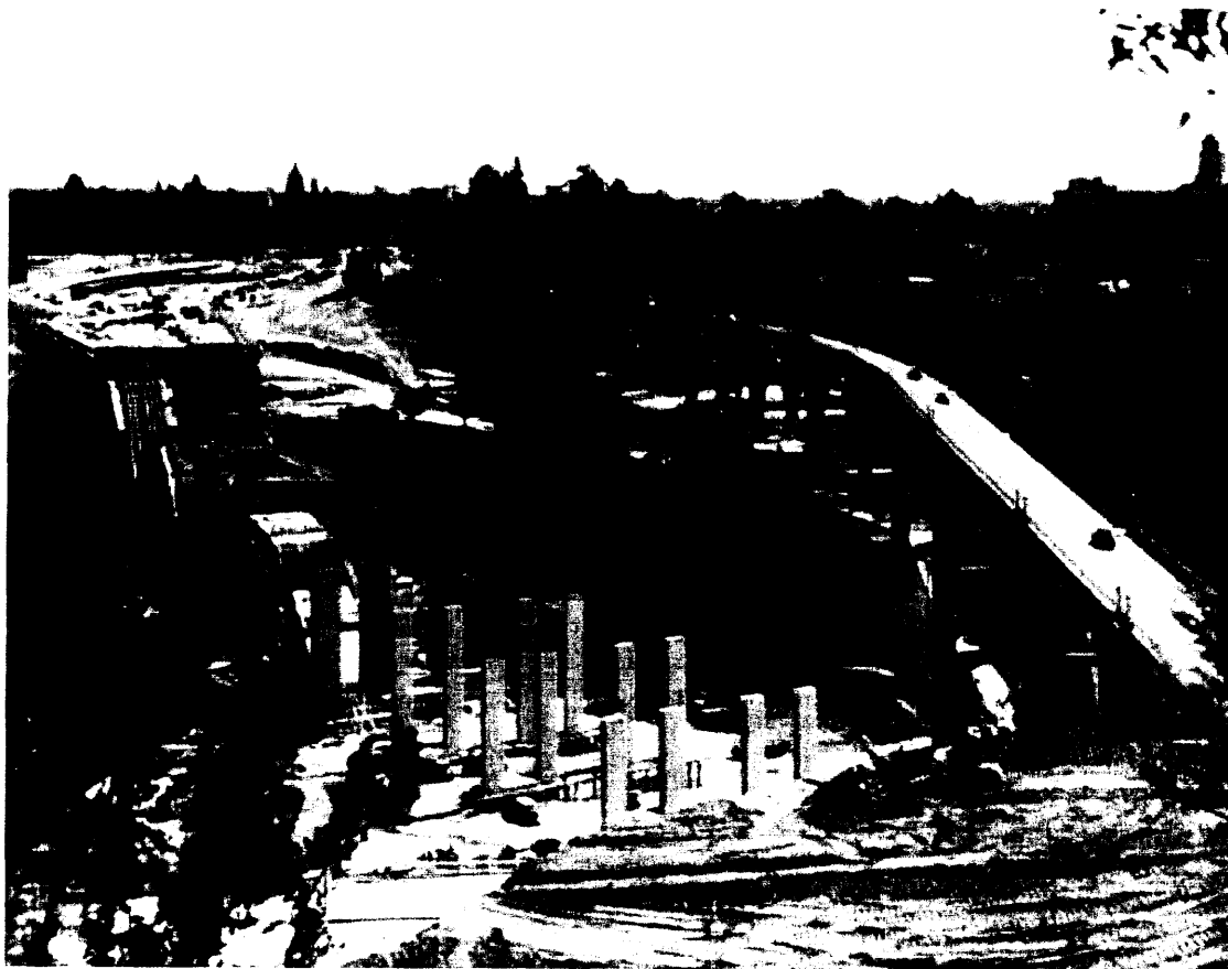
Pioneers Bridge under construction in 1951.
