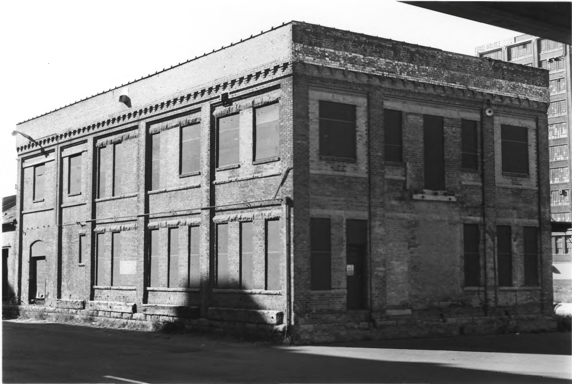
Minneapolis & St. Louis Railway Co. Freight Depot, Minneapolis Warehouse Historic District
