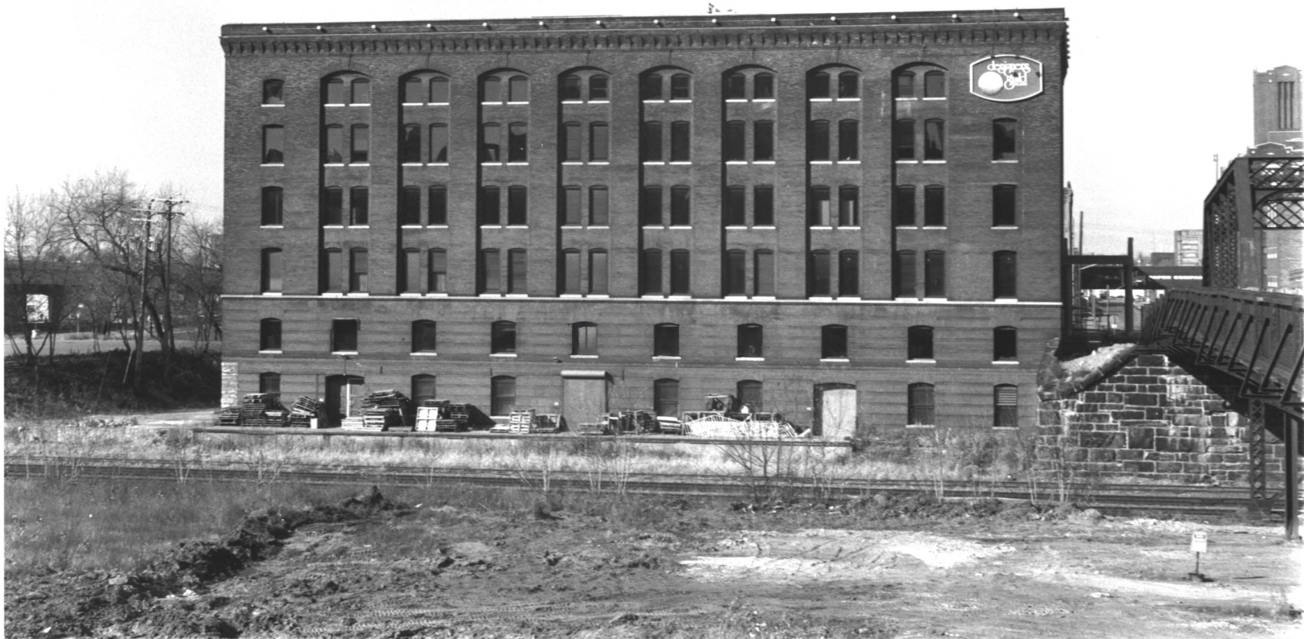
Minnesota Moline Plow Company, Minneapolis Warehouse Historic District
