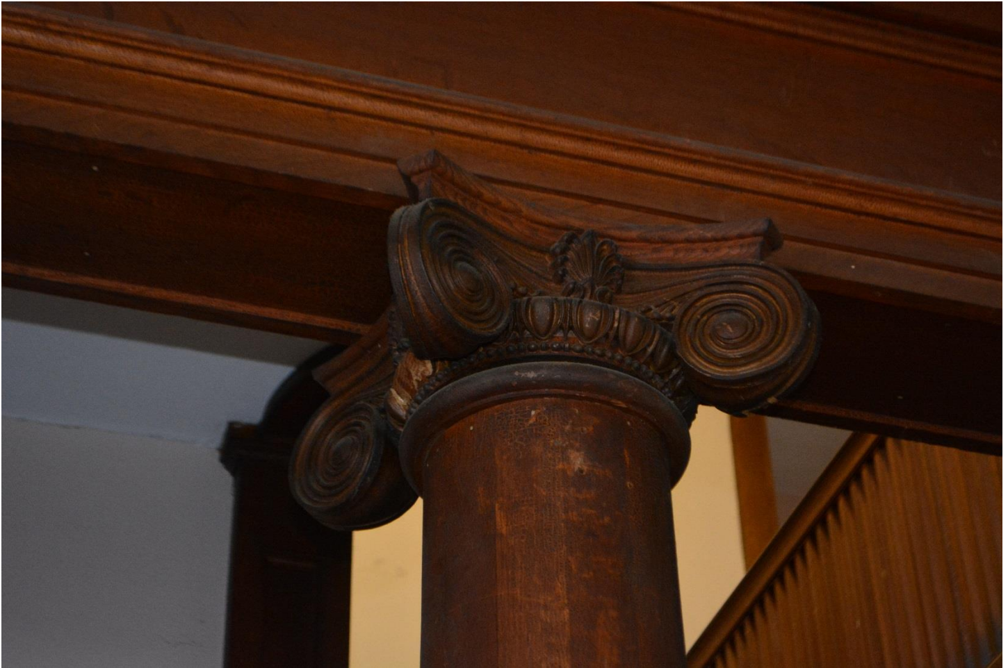
Photo 15 - Interior, first floor detail of column capitals in entry hall.
