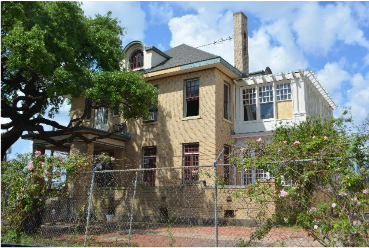
Photo 1 – South elevation and partial view east elevation, view northwest.
