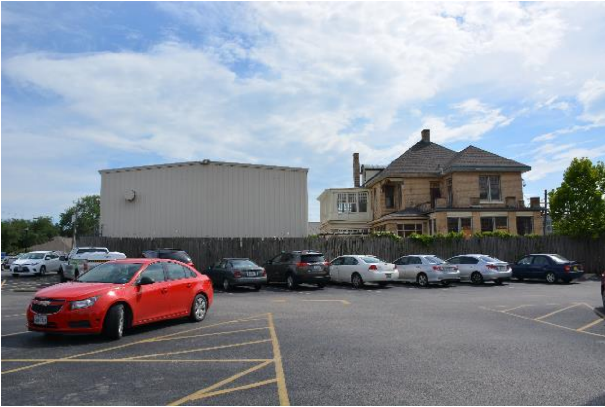
Photo 4 – North elevation (right) and non-contributing metal storage building (left), view south.
