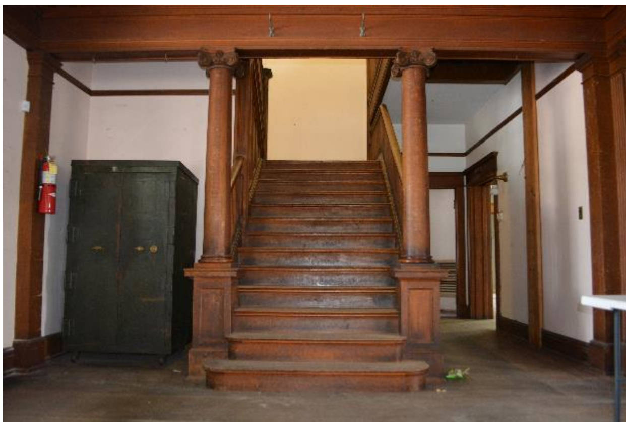
Photo 7 – Interior, first floor front entry hall and grand staircase, view north.
