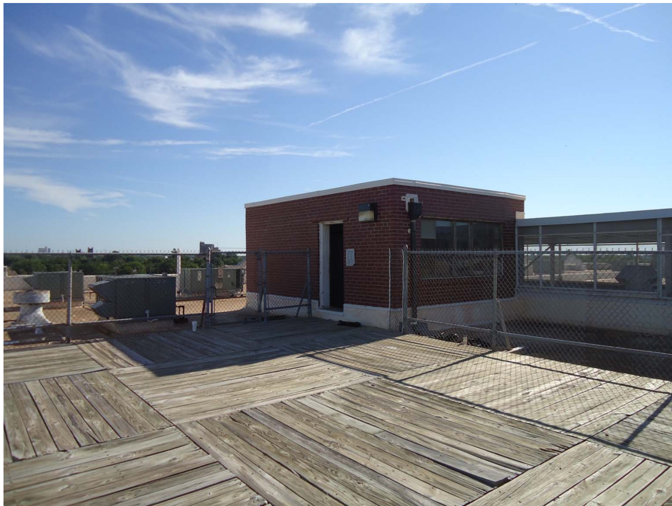
Photo 5 of 10. Headhouse/room that provides access to the roof. View northeast.
