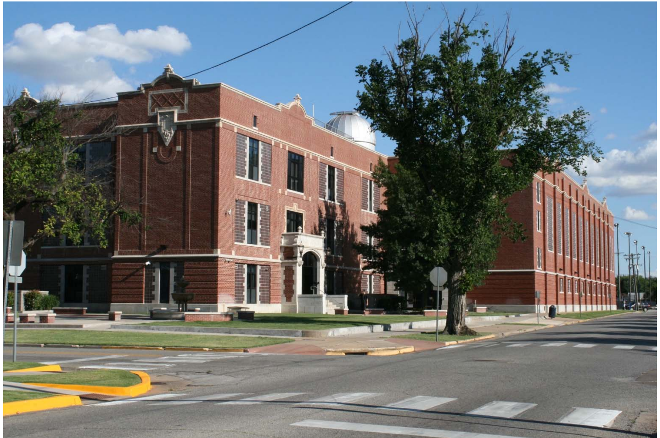
Photo 3 of 10. West elevation of Enid High School with view of EHS Observatory on roof. View southeast.
