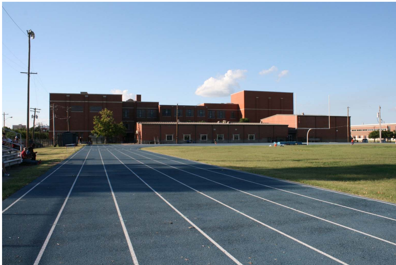
Photo 4 of 10. South elevation of Enid High School. View north.
