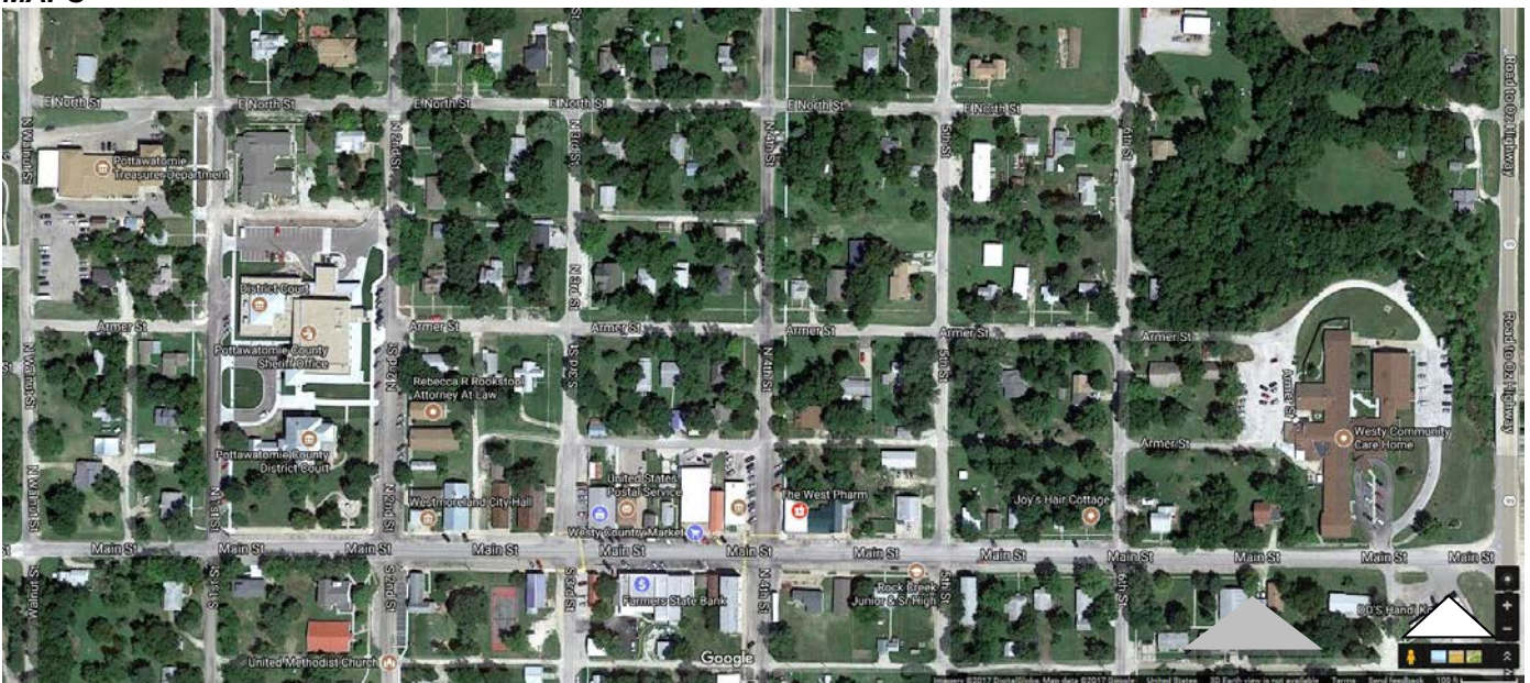
Figure 2 - Aerial View of Context - Town of Westmoreland, County Seat of Pottawatomie County.
