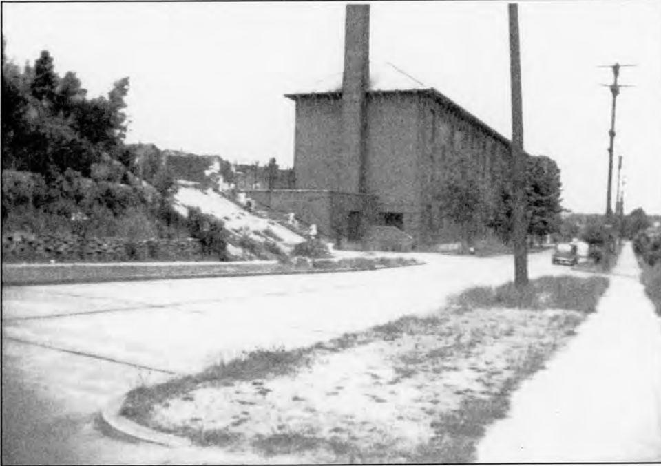
View looking north along Dayton Avenue North toward the 1918 building, showing south and east façades. Circa 1940, after the widening and paving of Dayton. (Unknown source, photo courtesy of Dale Reuterlinger.)
