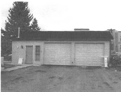
Modern Garage, south elevation (non-contributing)
