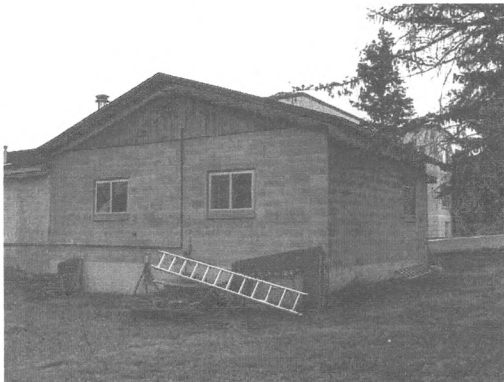
Concrete Garage, south and west elevations (non-contributing)
