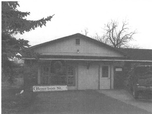
Concrete Garage, east elevation (non-contributing)
