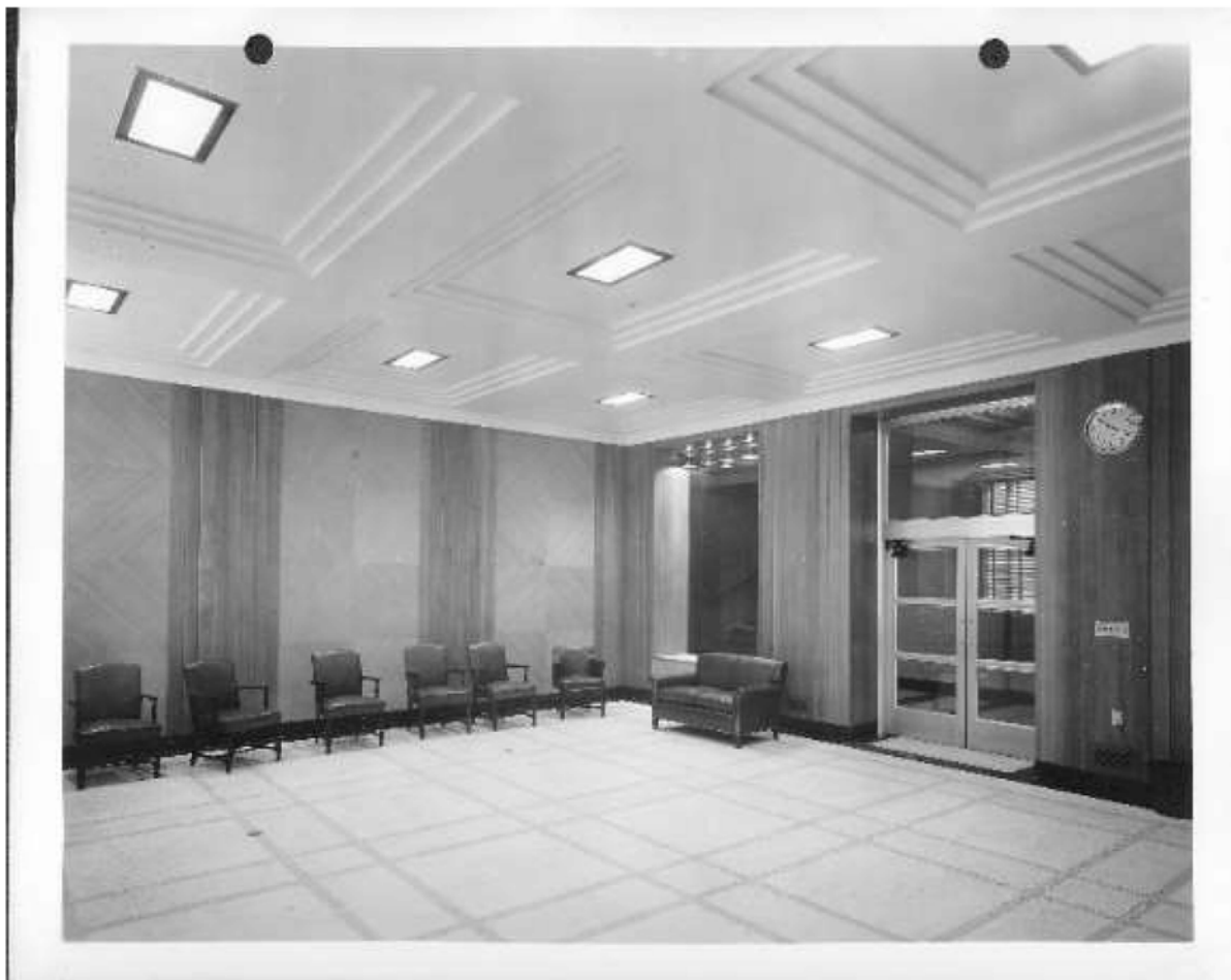
Figure 11: Exhibit Hall, 1939 (currently Room 200). Rodney Meadows, Motter & Meadows, Architects, archive.
