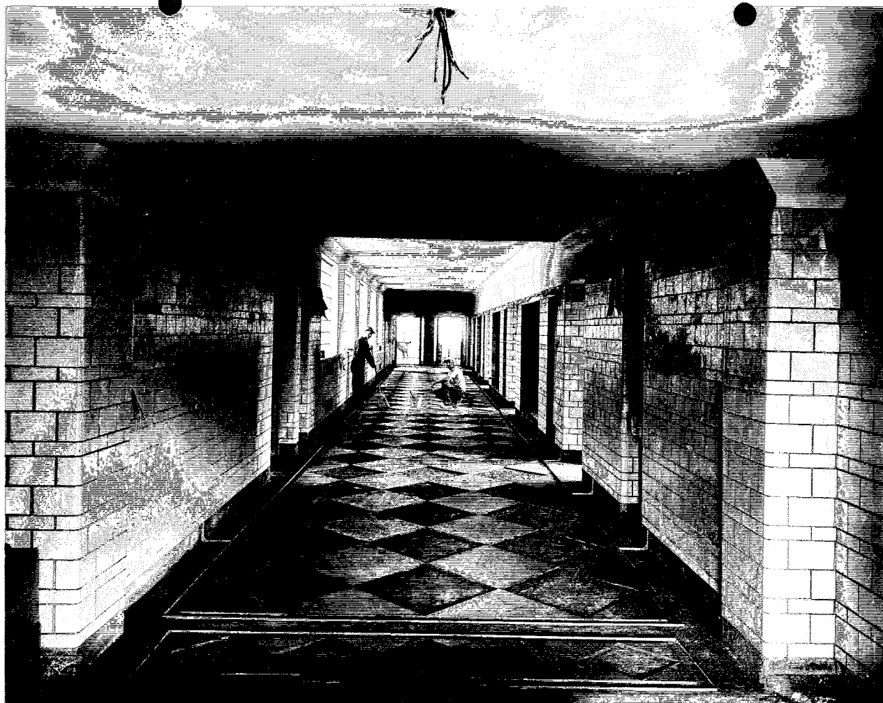
Figure 5: Terrazzo floor installation, third floor hall, 1939. Rodney Meadows, Motter & Meadows,
