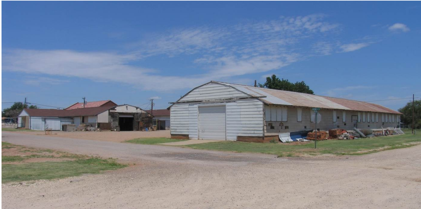
Photo 24 Childress ISD Maintenance Buildings, Avenug G (#83-85)
