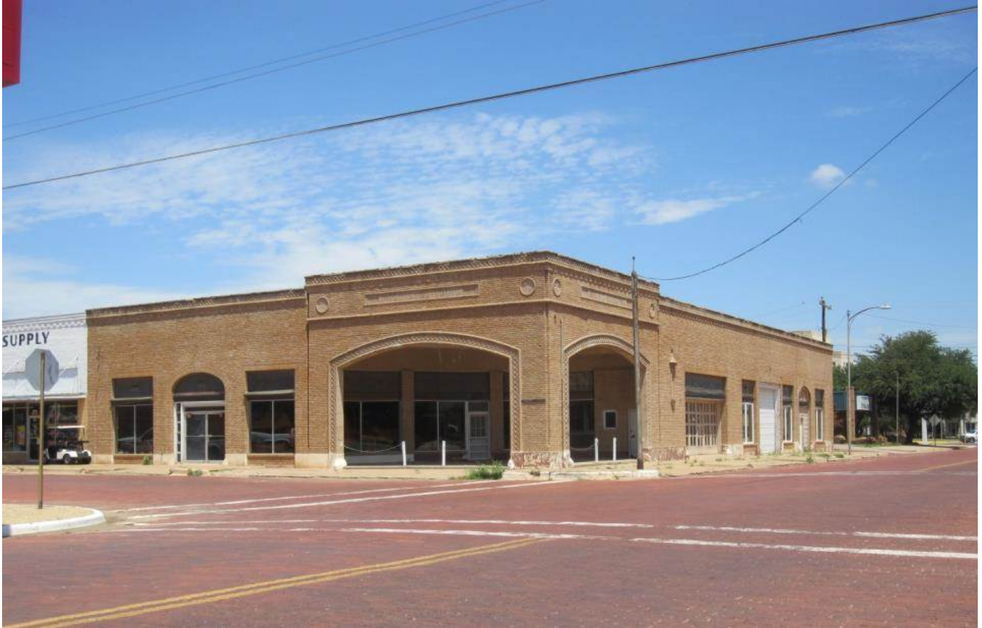
Photo 20 Michie Building, 401 Main (#123)
