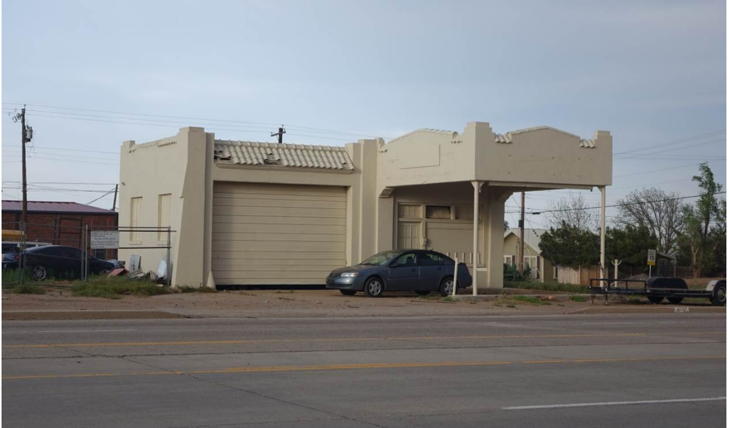
Photo 15 100 Avenue F NW (#66)
