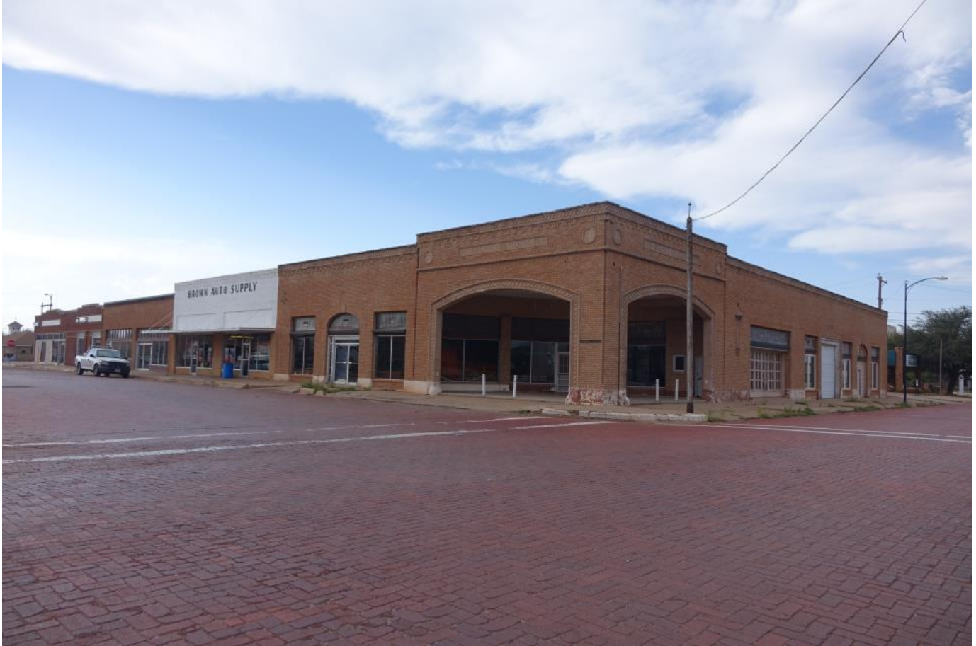
Photo 4 Avenue D at Main, facing northwest
