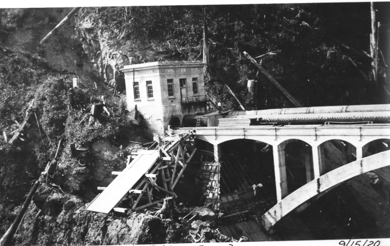
East Abut. Concrete Bridge Comp 2
