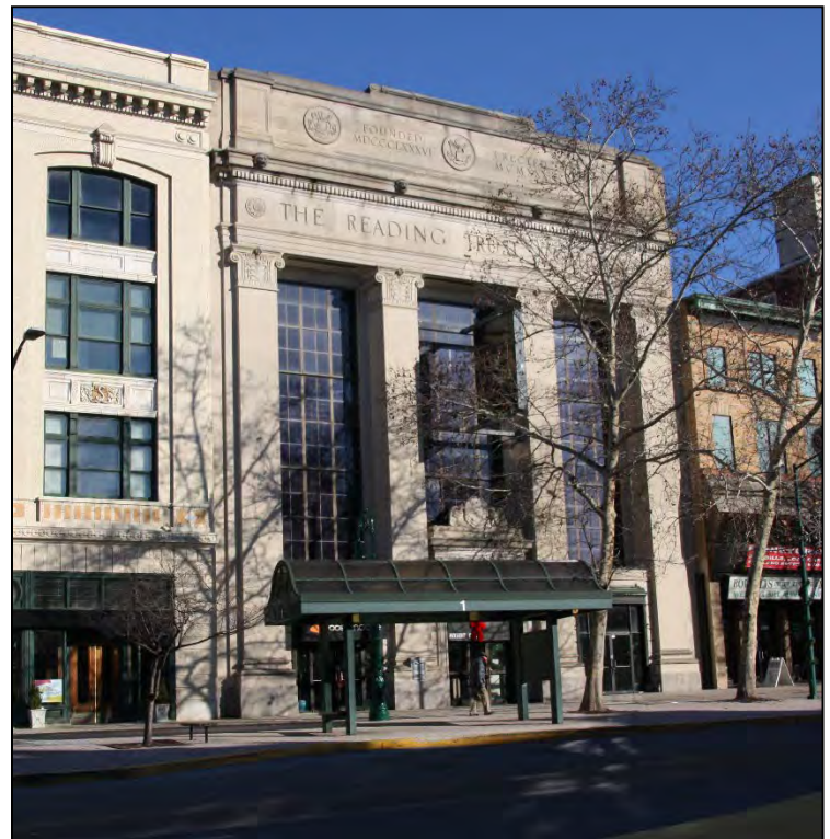
FIGURE 21 – Reading Trust Company, 511 Penn Street, Reading, www.bing.com/maps , accessed September 15, 2013.
