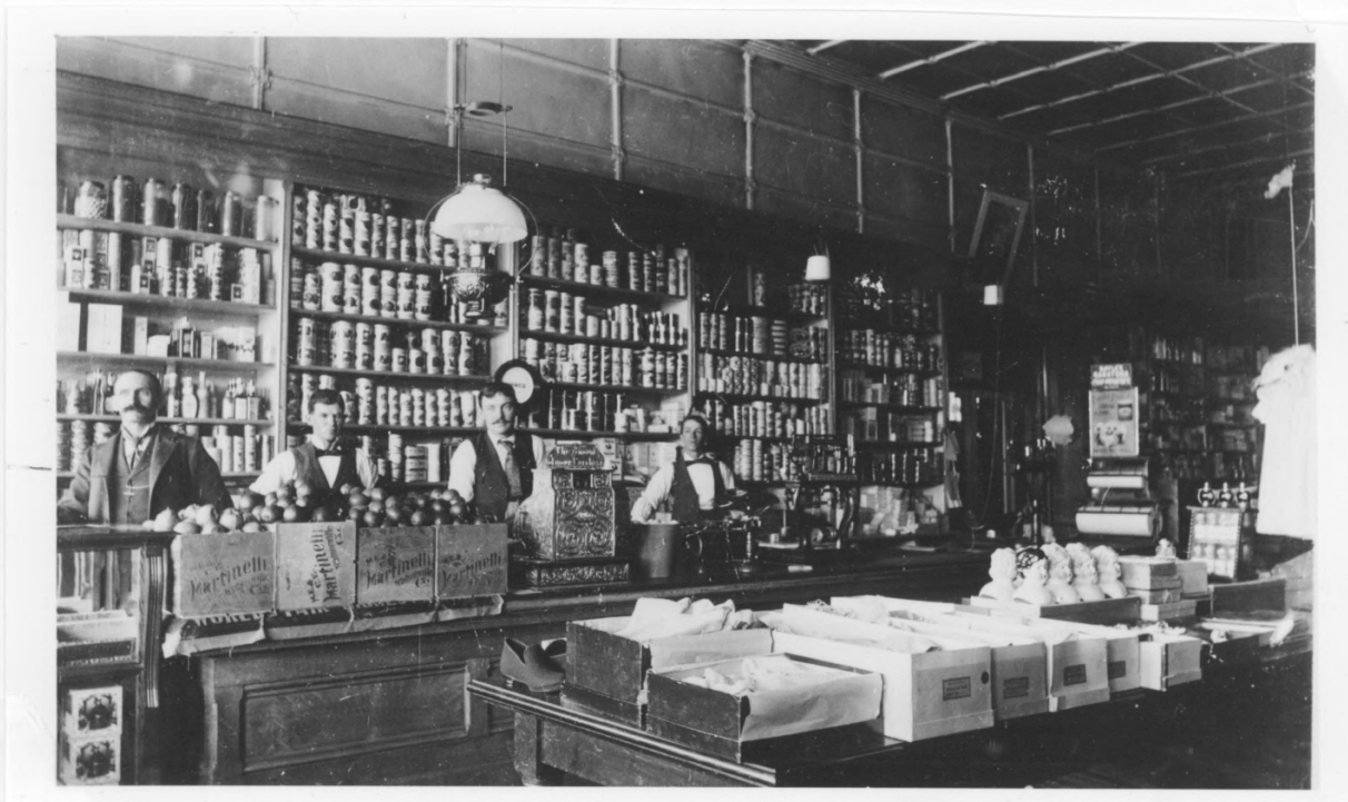
J. I. GARDNER'S STORE-HISTORIC PHOTO Sharlot Hall Museum Archives Bu-I-111PC (north wall interior)
