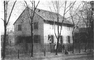
1869 view of the building taken prior to the construction of the first major addition showing the west (gable end) and south elevations of the 1739 sections.
