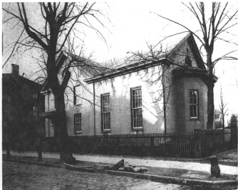
View of the building in 1874 after the construction of the first addition showing the south and east elevations.
