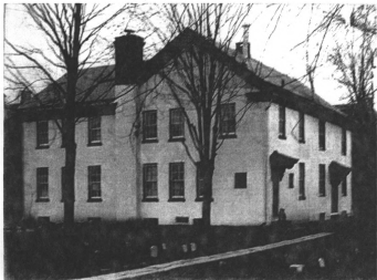
Undated photograph of the north and west elevations showing the 1896 addition at left and the 1874 addition at right (gable end section of north elevation and all of west elevation).
