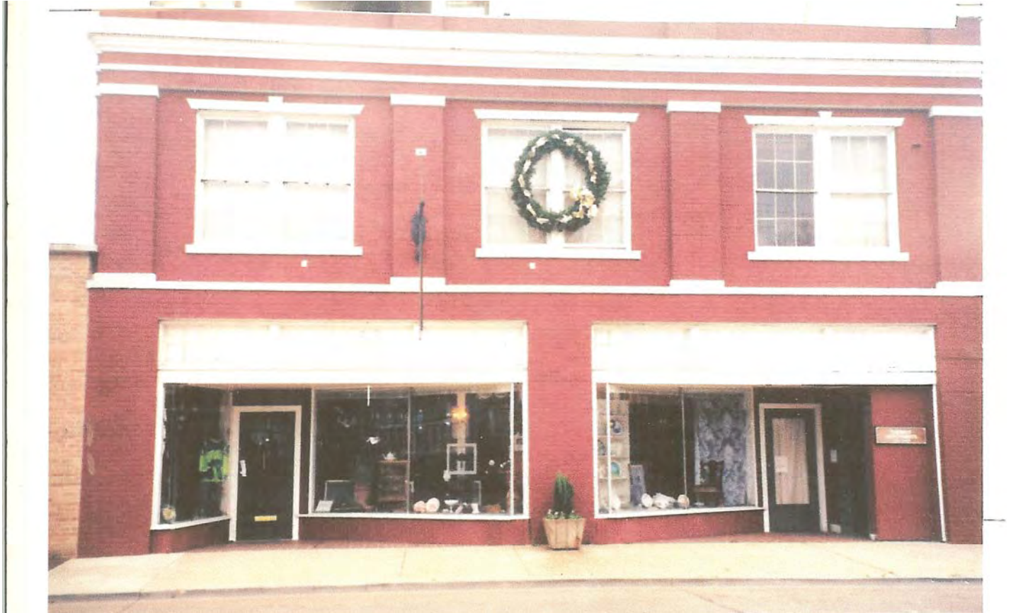
Figure 15. Photo of the building in 2004 prior to the storefront rehabilitation showing the altered c. 1948 storefront. Image courtesy of the author.
