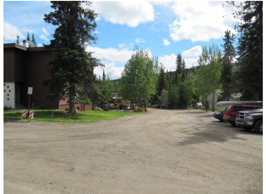
2 of 16. Boiler House Spur Road.
