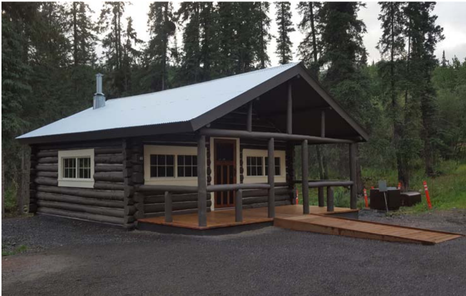
4 of 16. Building 22 (Office Building).
