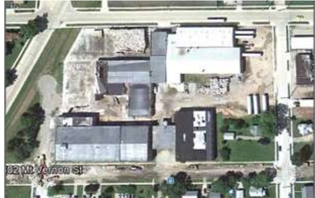
Figure 8: 2011 aerial view after demolition (2 buildings).
