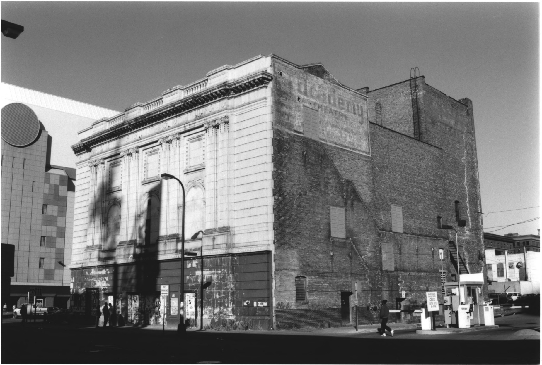
Sam S. Shubert Theatre 22 Seventh Street North, Minneapolis Hennepin Co, MN 012456-15
