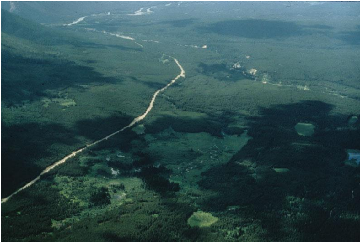
Figure #2: Aerial photograph of the completed Camas Creek Road, 1967.
