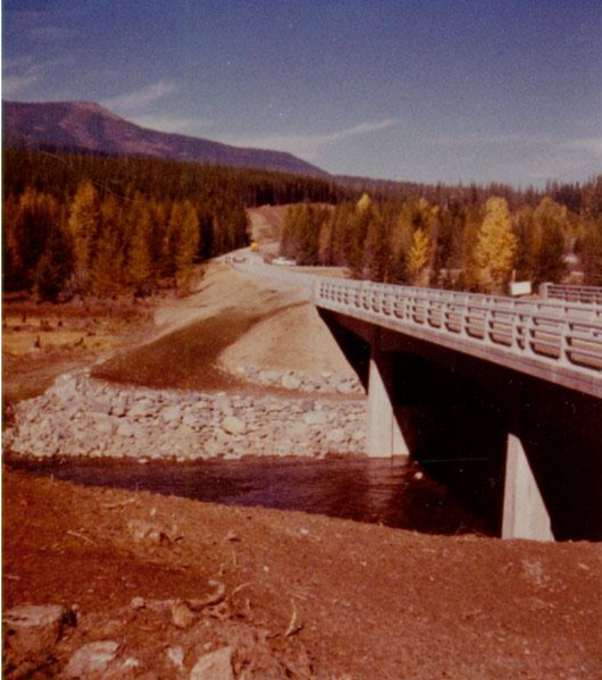
Figure #4: McDonald Creek Bridge, soon after completion.
