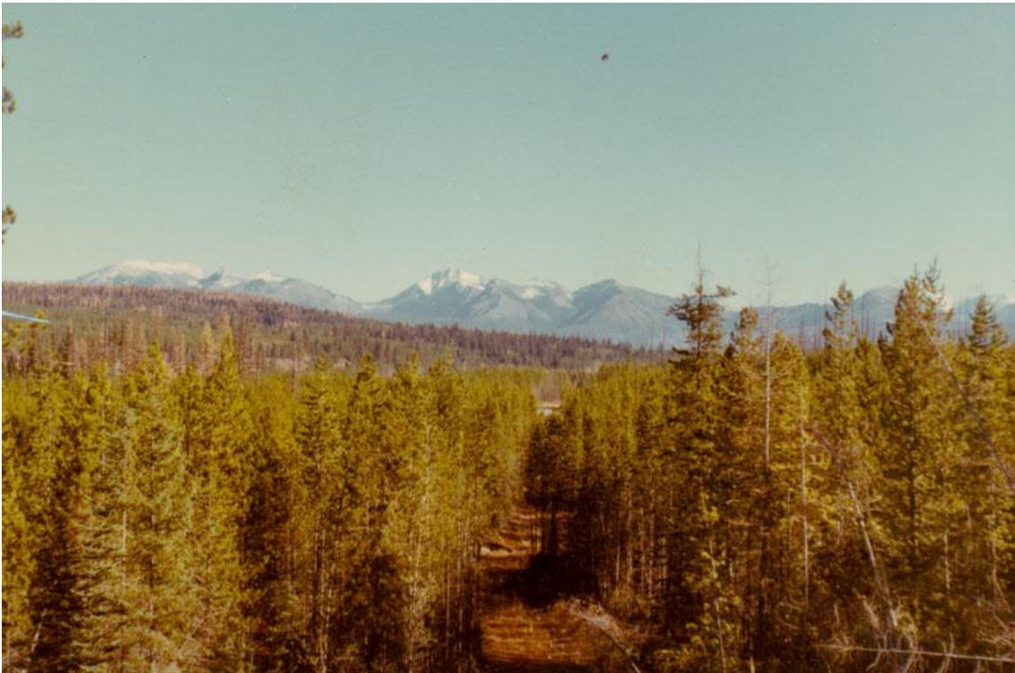
Figure #1: Pioneering/clearing work for the Camas Road.
