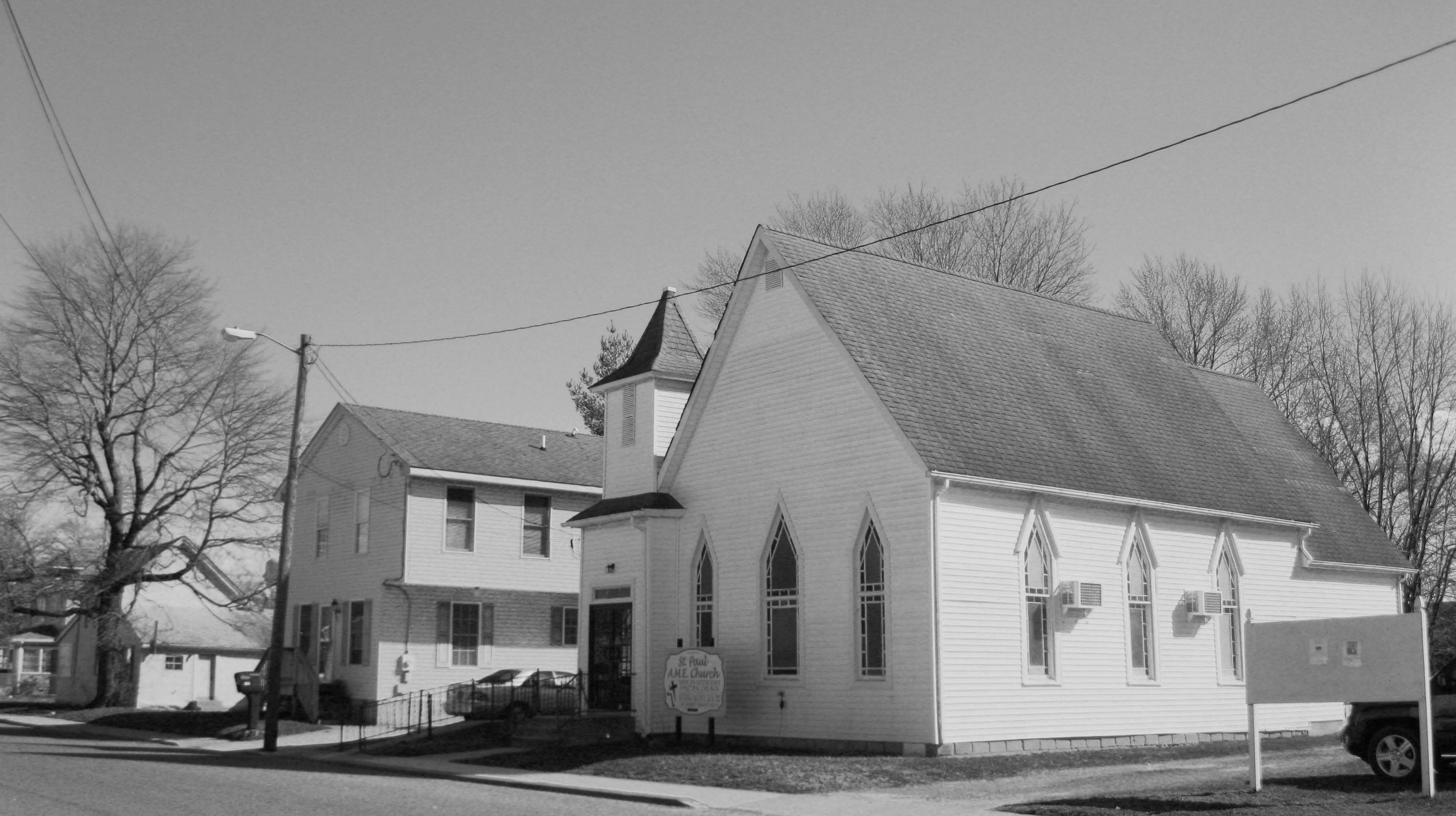
DE_Kent County_St. Paul A.M.E. Church Three-quarter view of church with neighboring dwellings east of church along West Mispillion Street 02 of 13
