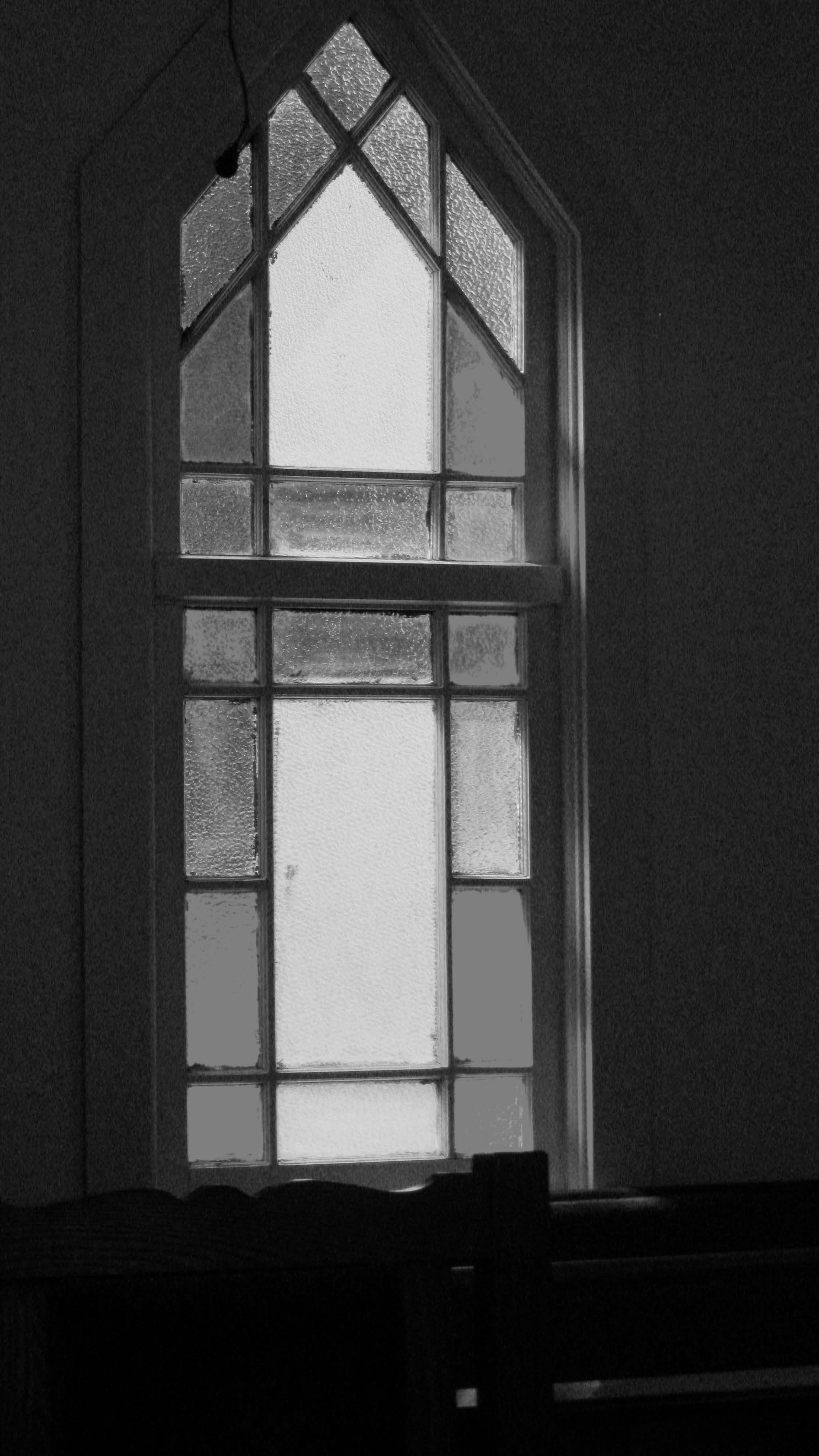
DE_Kent County_ St. Paul A.M.E. Church Stained glass window added c. 1948 04 of 13
