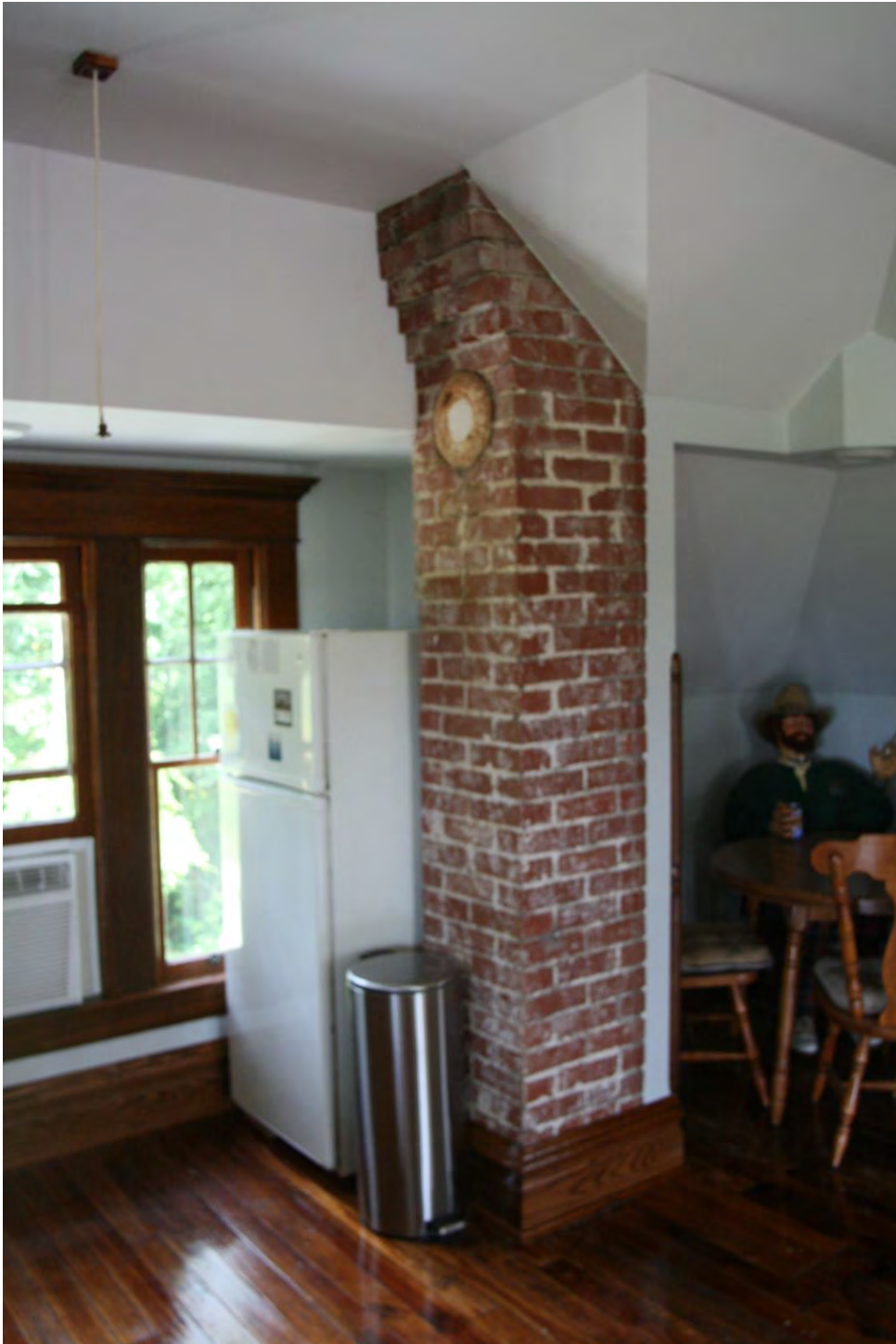
Photo 28: Interior, Carriage house, second floor gentlemen's club, northwest corner
