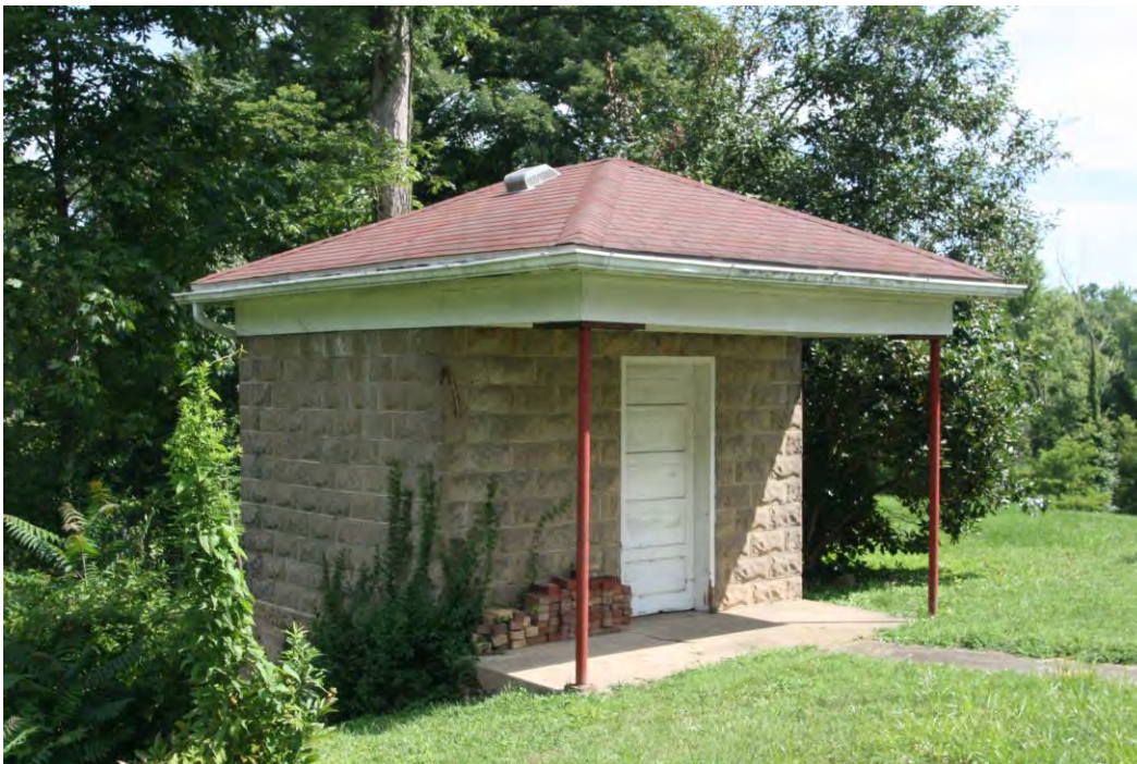
Photo 10: Smokehouse, southwest corner, facing northeast
