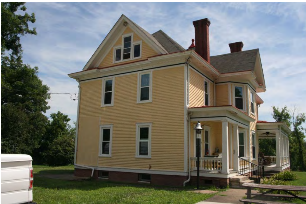
Photo 4: Main house, west elevation, facing east
