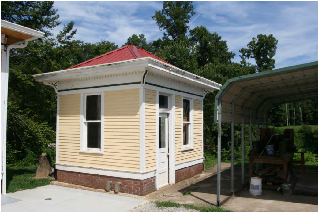
Photo 8: Well and Generator building, southeast corner, facing northwest
