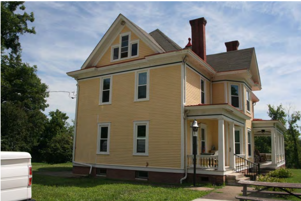
Photo 4: Main house, west elevation, facing east
