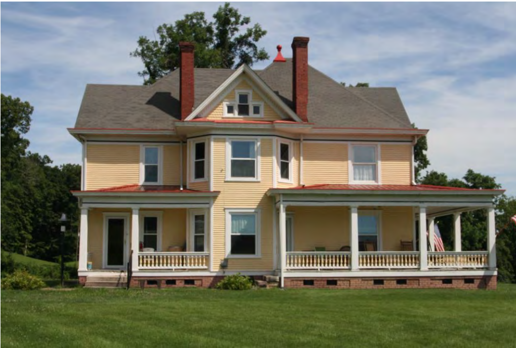
Photo 5: Main house, south elevation, facing north
