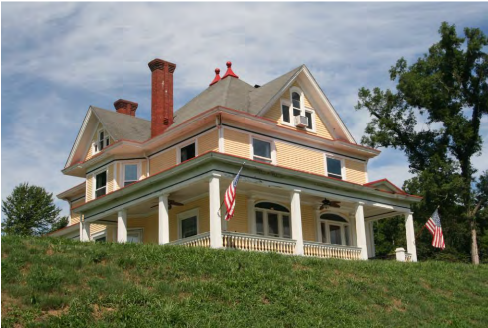
Photo 1: Main house, southeast corner of house, facing northwest
