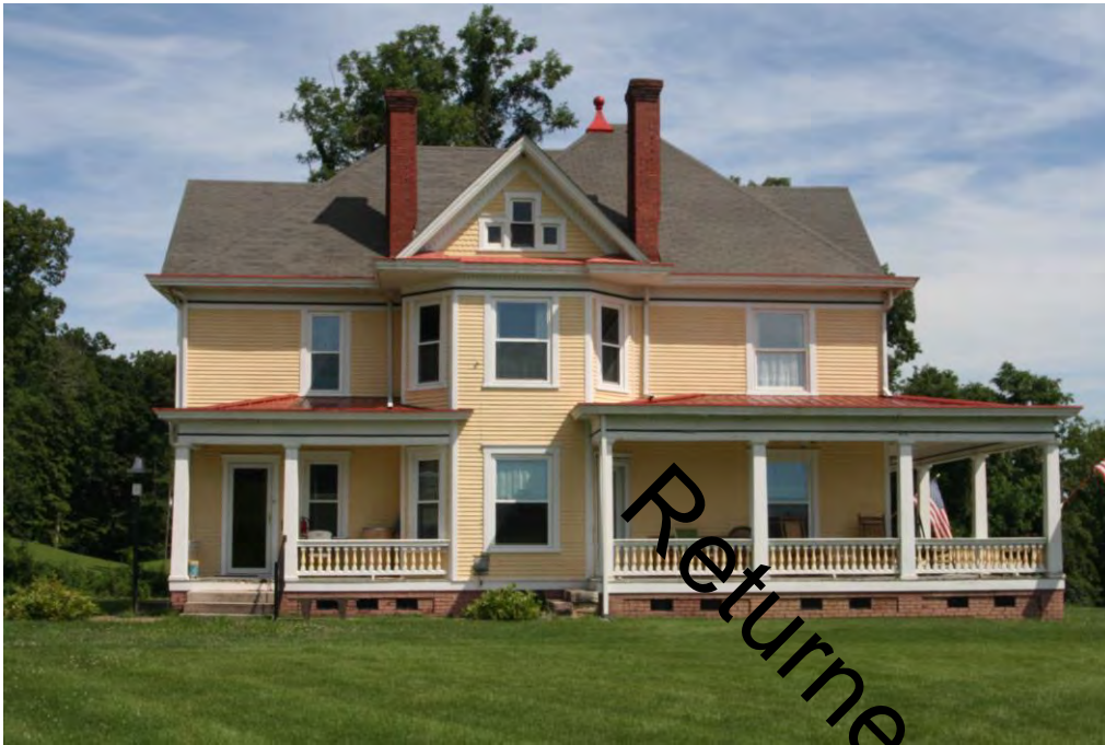
Photo 5: Main house, south elevation, facing north
