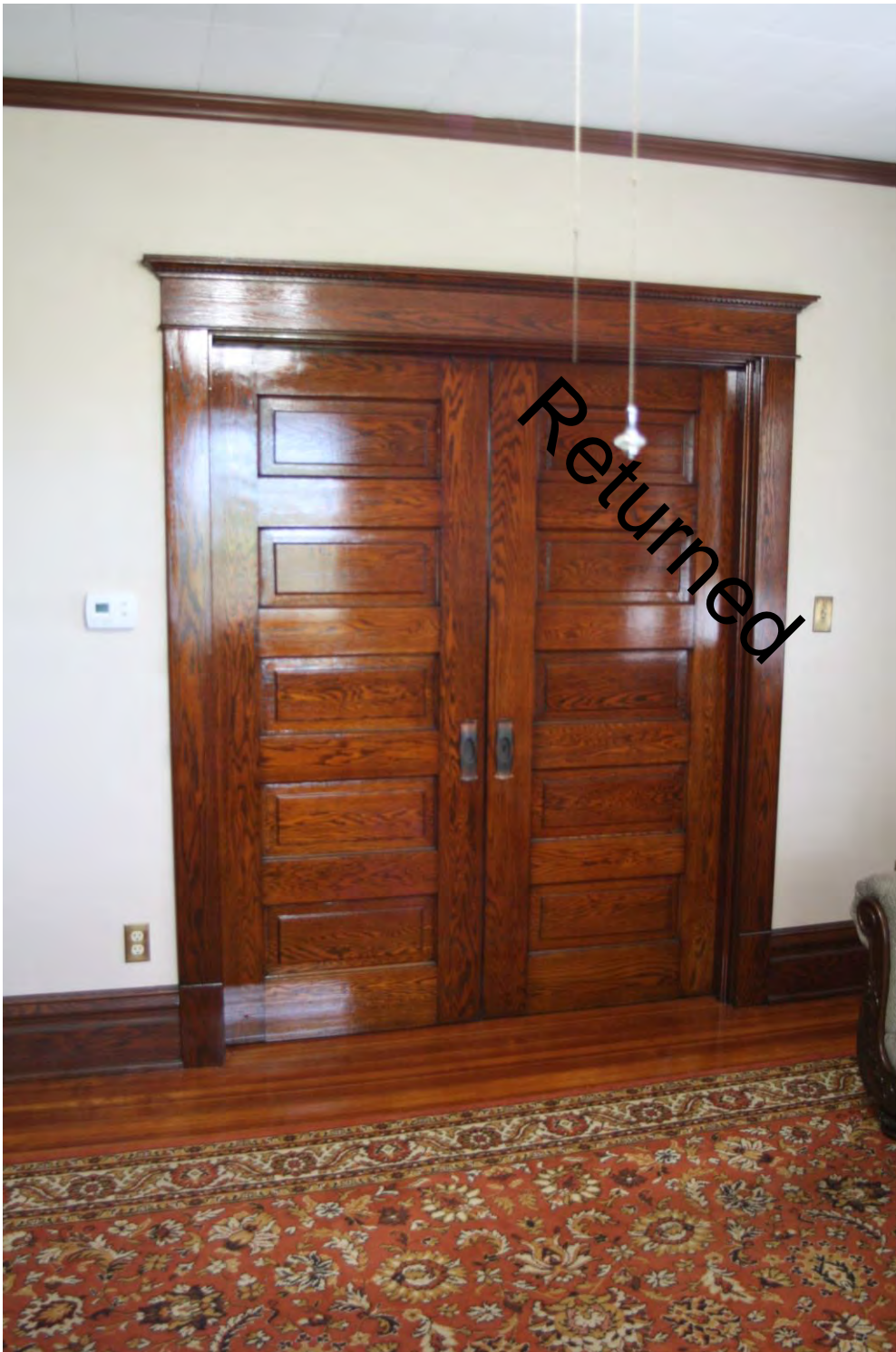
Photo 13A: Interior, Pocket door between foyer and parlor, taken from foyer
