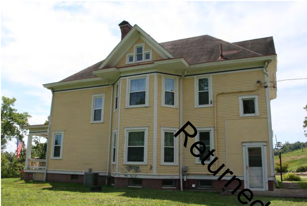
Photo 3: Main house, north elevation, facing south, shows entry to basement
