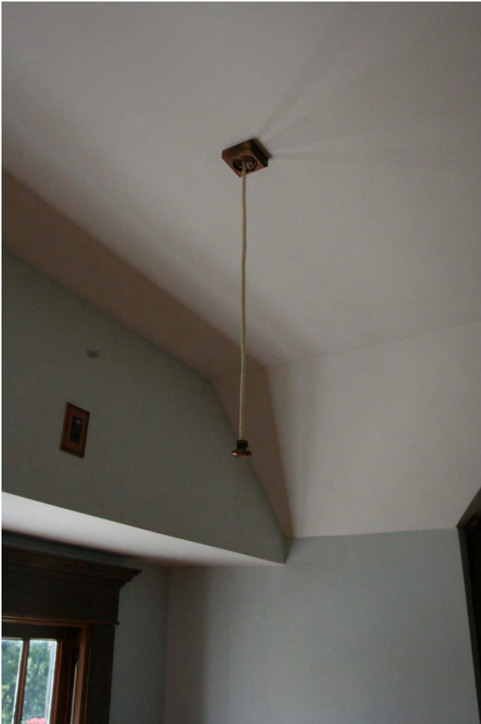
Photo 29: Interior, Carriage house, pullcord for ventilation system in dormers
