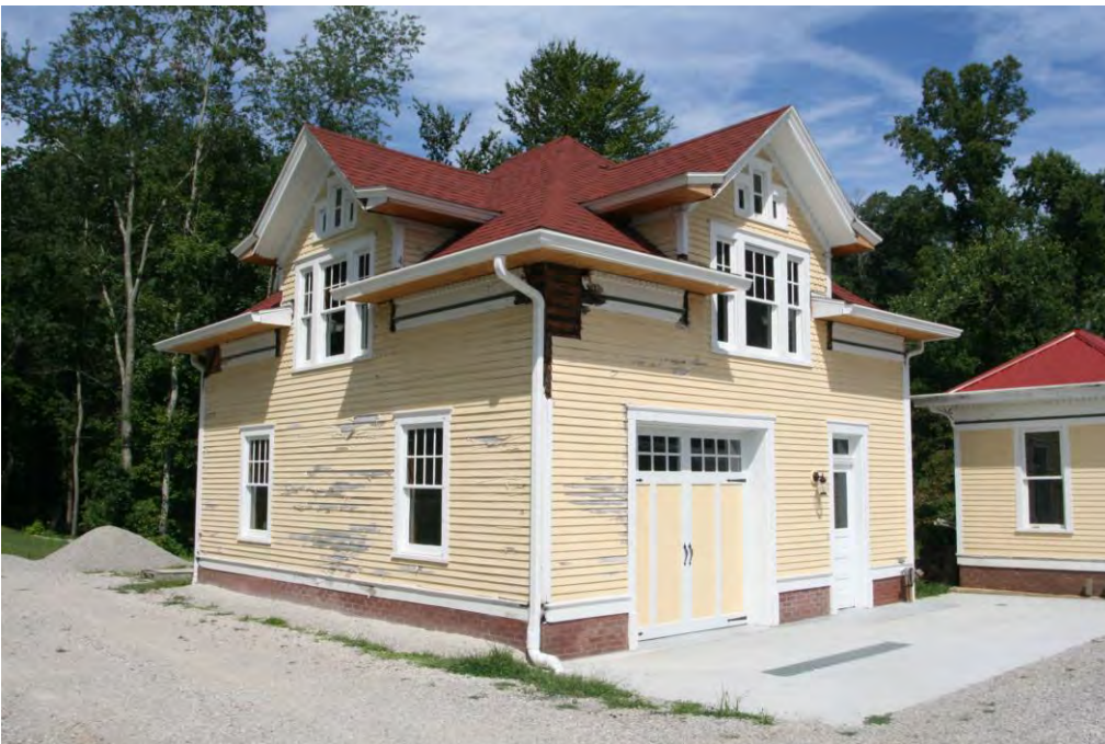
Photo 6: Carriage House, southeast corner, facing northwest
