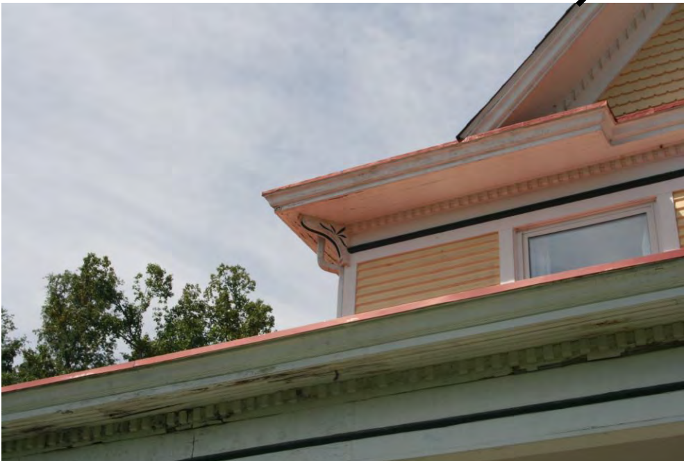
Photo 1A: Main house, decorative bracket on southwest corner of south elevation, facing northwest
