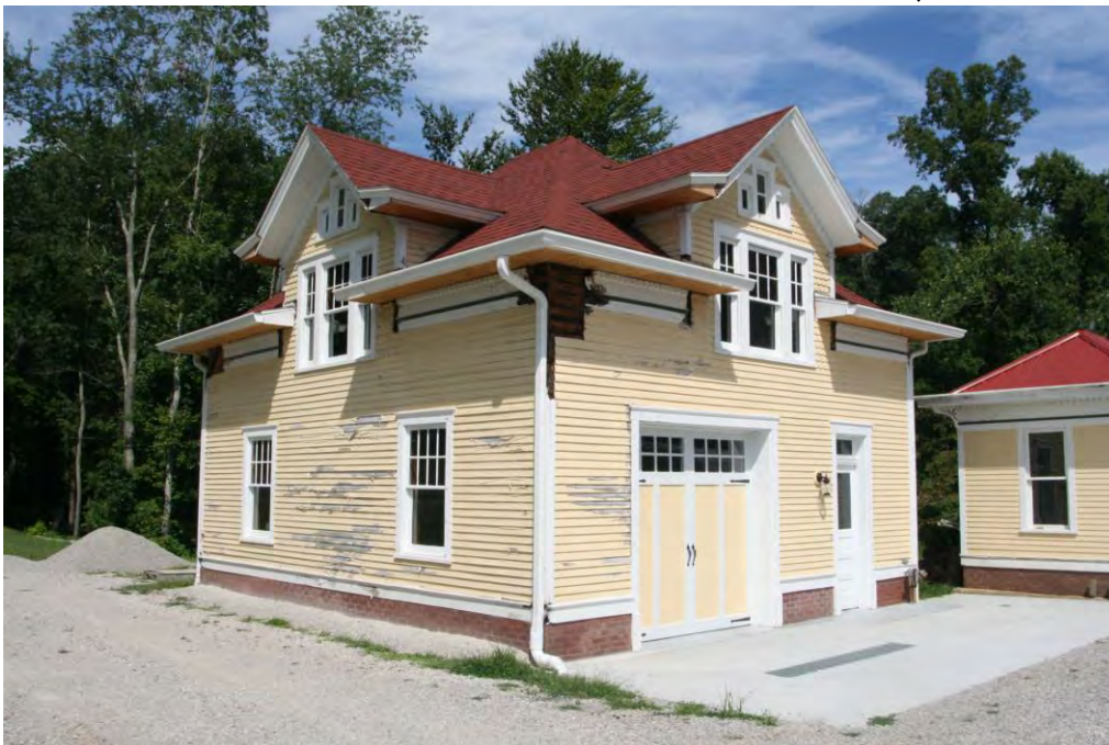
Photo 6: Carriage House, southeast corner, facing northwest
