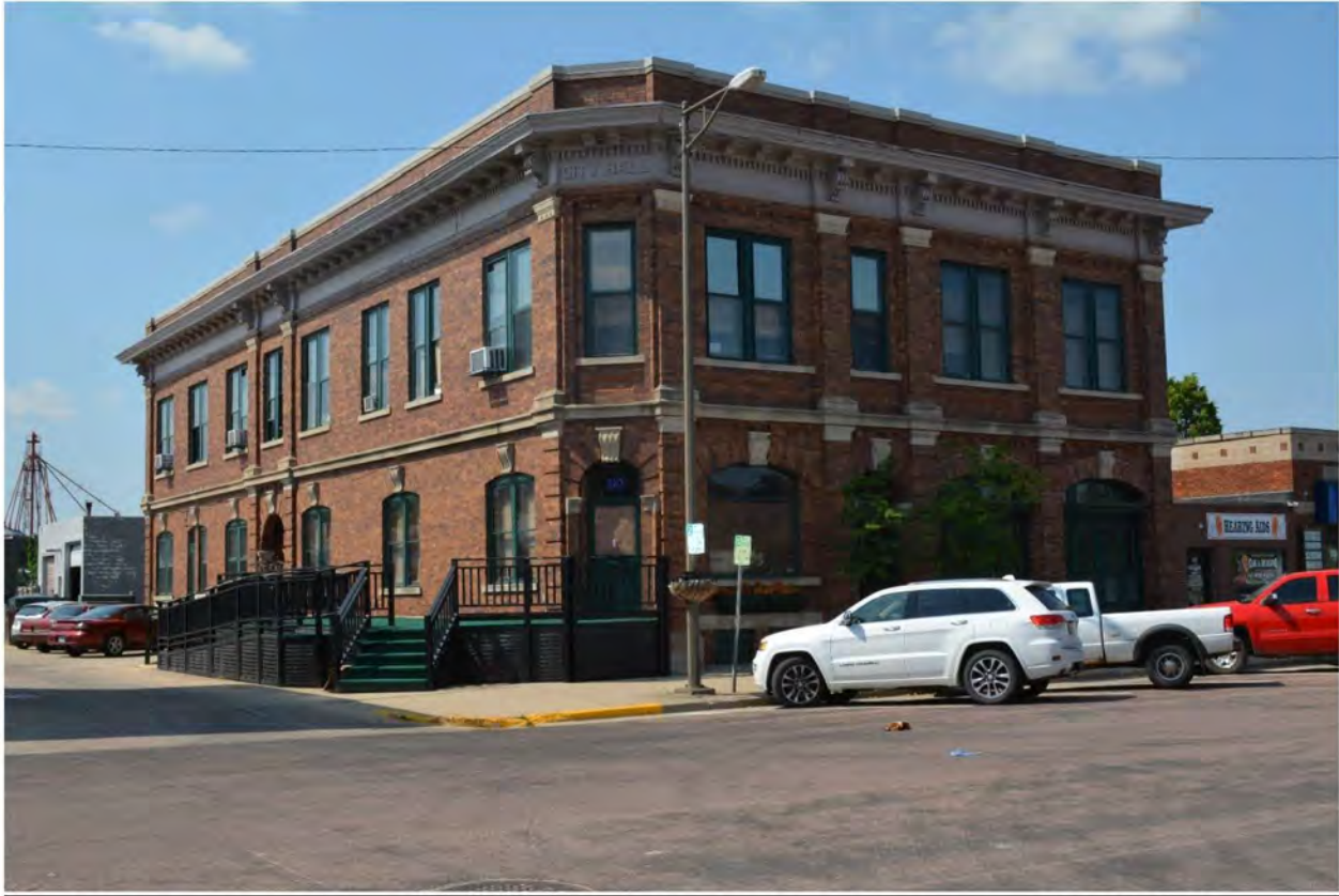
SD_BrookingsCounty_BrookingsCommercialHistoricDistrictAmendment2020_0015 Looking SW at 310 4 th Street.
