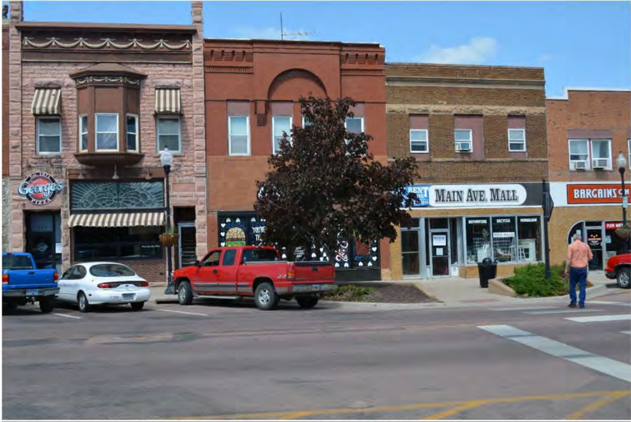
SD_BrookingsCounty_BrookingsCommercialHistoricDistrictAmendment2020_0039 Looking W at 313 Main (center with brick arch).
