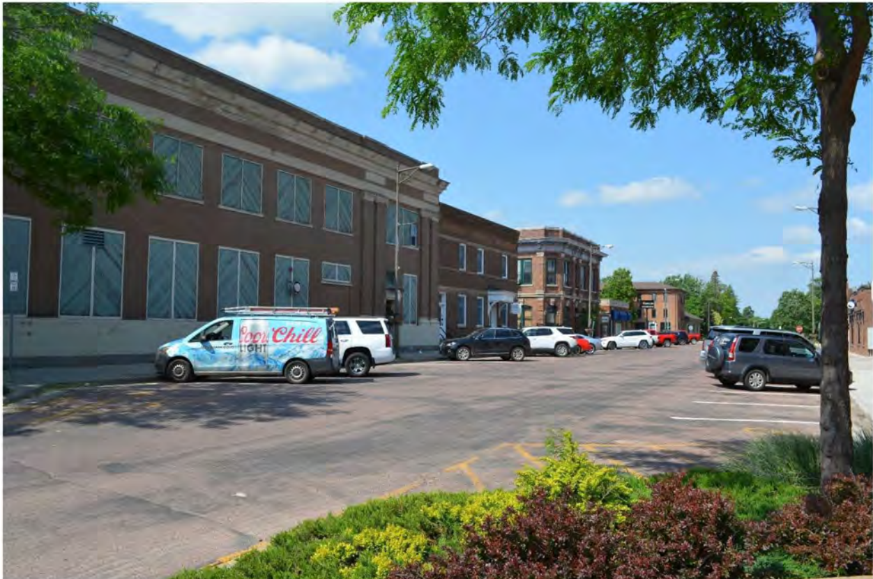
SD_BrookingsCounty_BrookingsCommercialHistoricDistrictAmendment2020_0053 Looking SW at 327 Main and 316 and 310 4 th Street.
