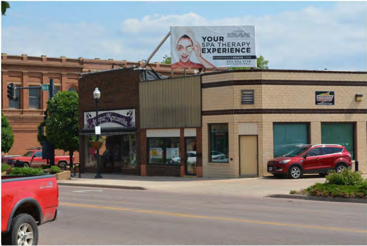
SD_BrookingsCounty_BrookingsCommercialHistoricDistrictAmendment2020_0032 Looking NE at 222, 224, and 226 Main (right to left).
