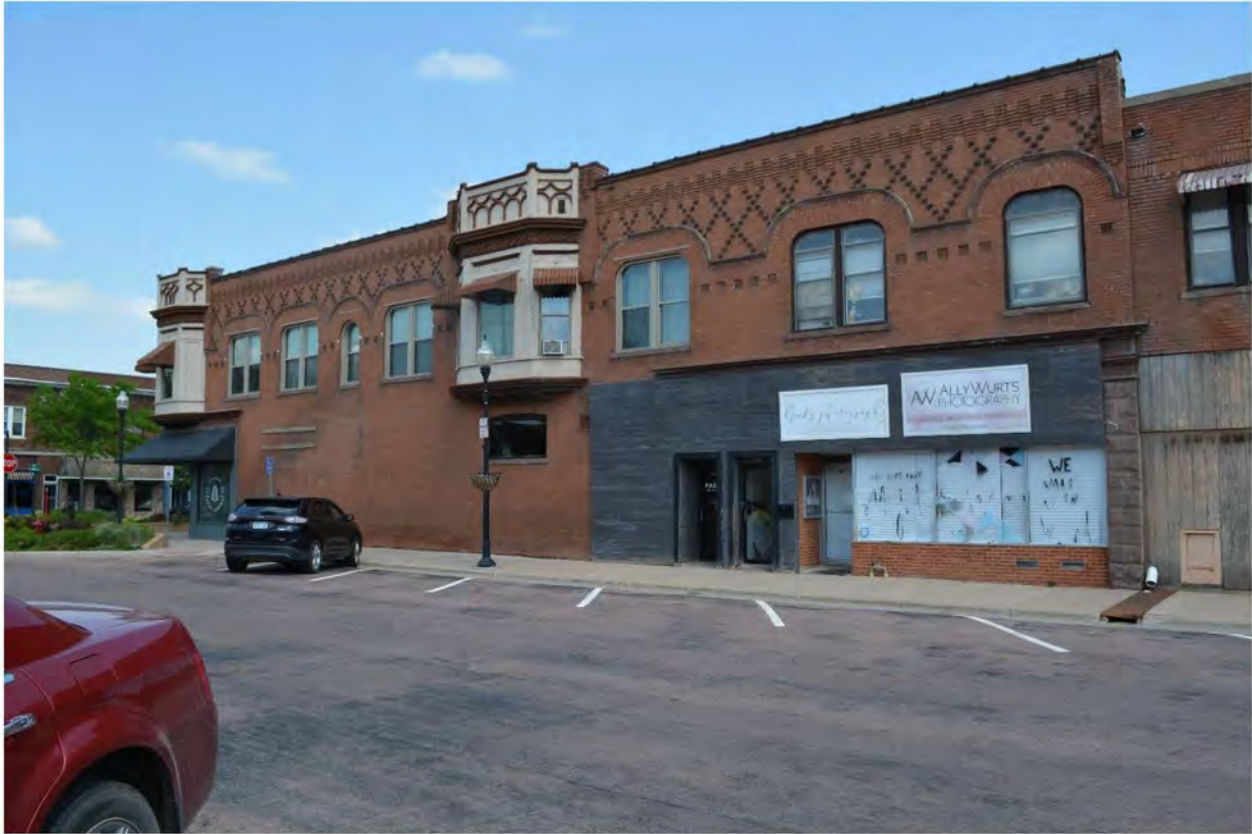
SD_BrookingsCounty_BrookingsCommercialHistoricDistrictAmendment2020_0044 Looking NW at 400-402 Main.
