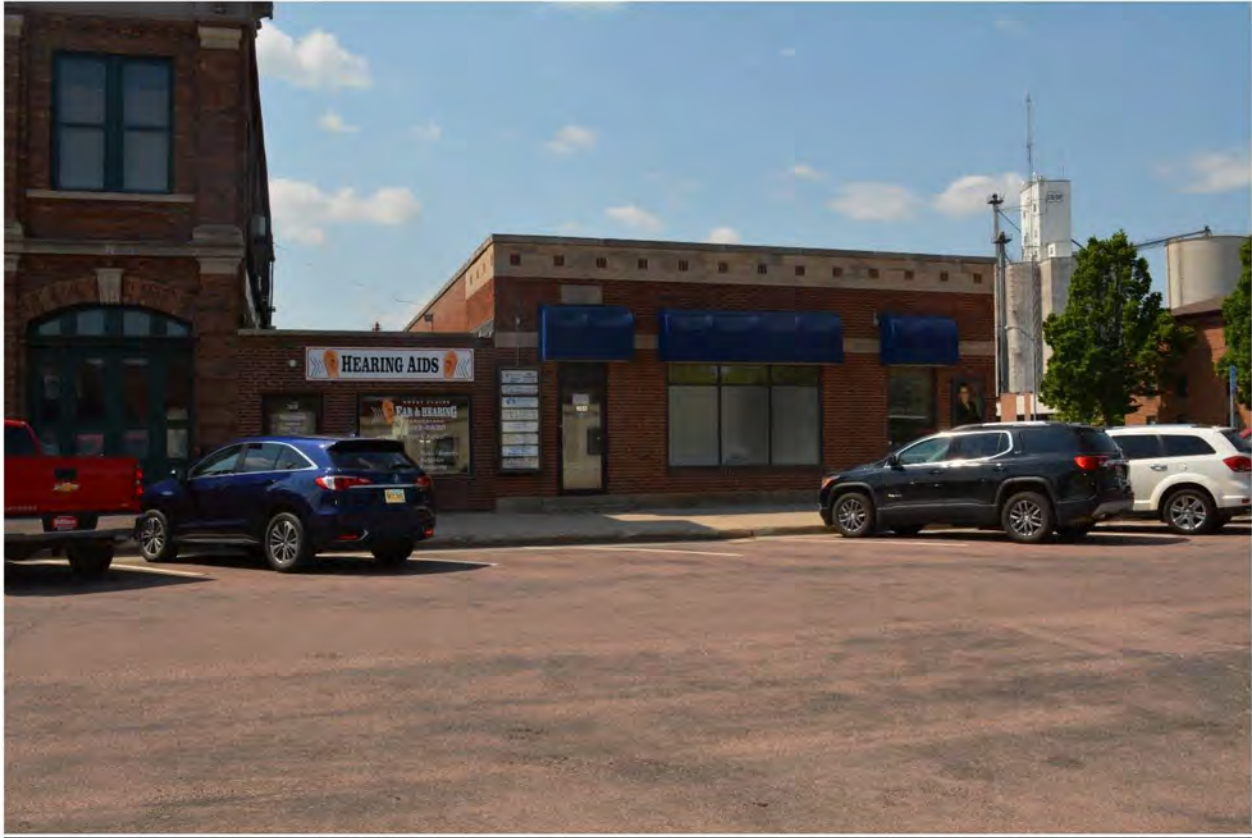
SD_BrookingsCounty_BrookingsCommercialHistoricDistrictAmendment2020_0016 Looking SW at 306 (right) and 308 (left) Main.
