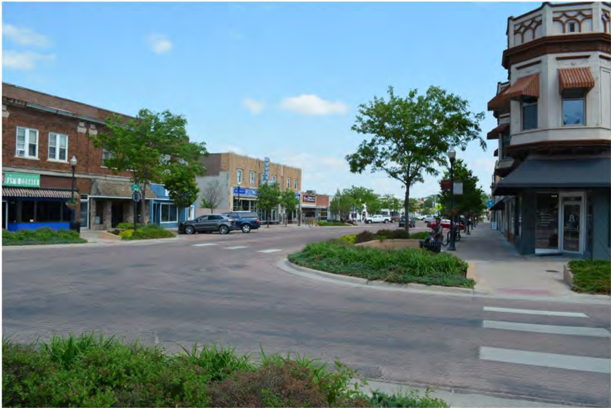
SD_BrookingsCounty_BrookingsCommercialHistoricDistrictAmendment2020_0058 Looking NW at the west side of 400 Block of Main.
