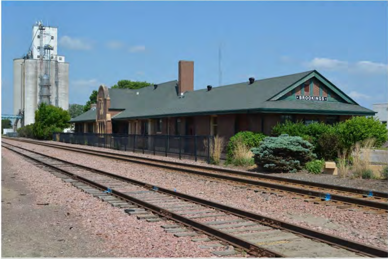
SD_BrookingsCounty_BrookingsCommercialHistoricDistrictAmendment2020_0030 Looking NW at 111 Main.
