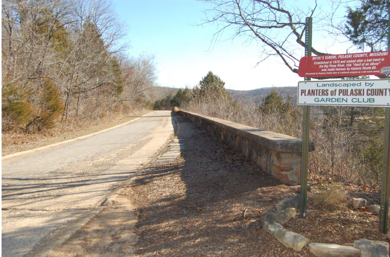
Figure 8. West of Devil's Elbow Historic District, along the original Route 66 alignment, this scenic overlook and stone wall were constructed by the Works Progress Administration (Photo: Ruth Keenoy; Source: Primas, Route 66 in Pulaski County , 64).
