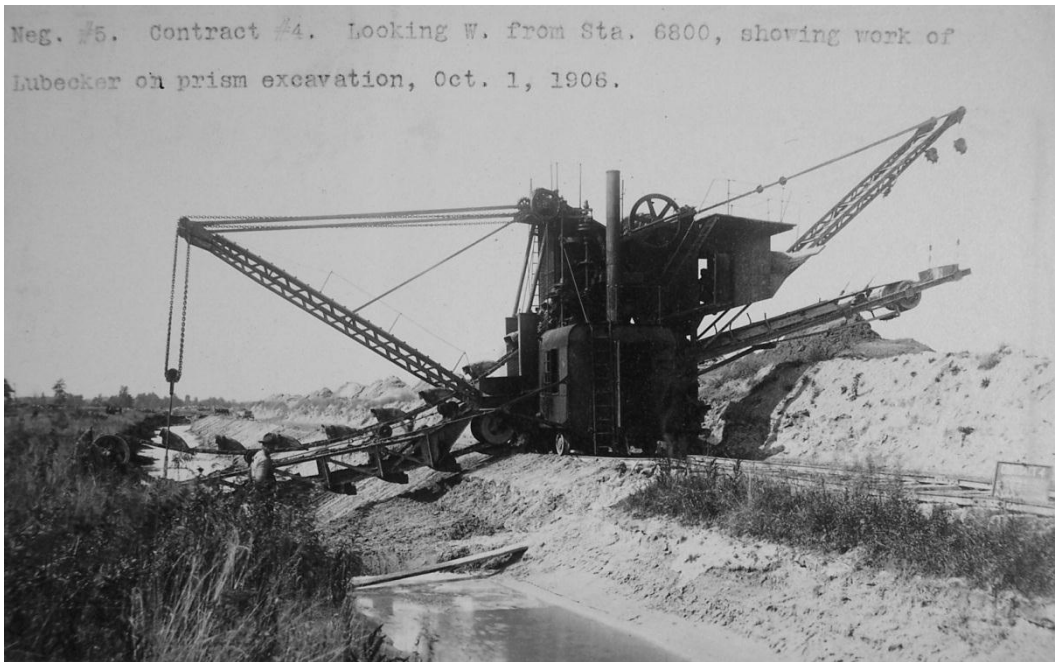
Figure 7 – Erie Canal, Lubecker Machine, used to widen existing channels, near Sylvan Beach, Oneida County, October 1, 1906 (Contract 4)
