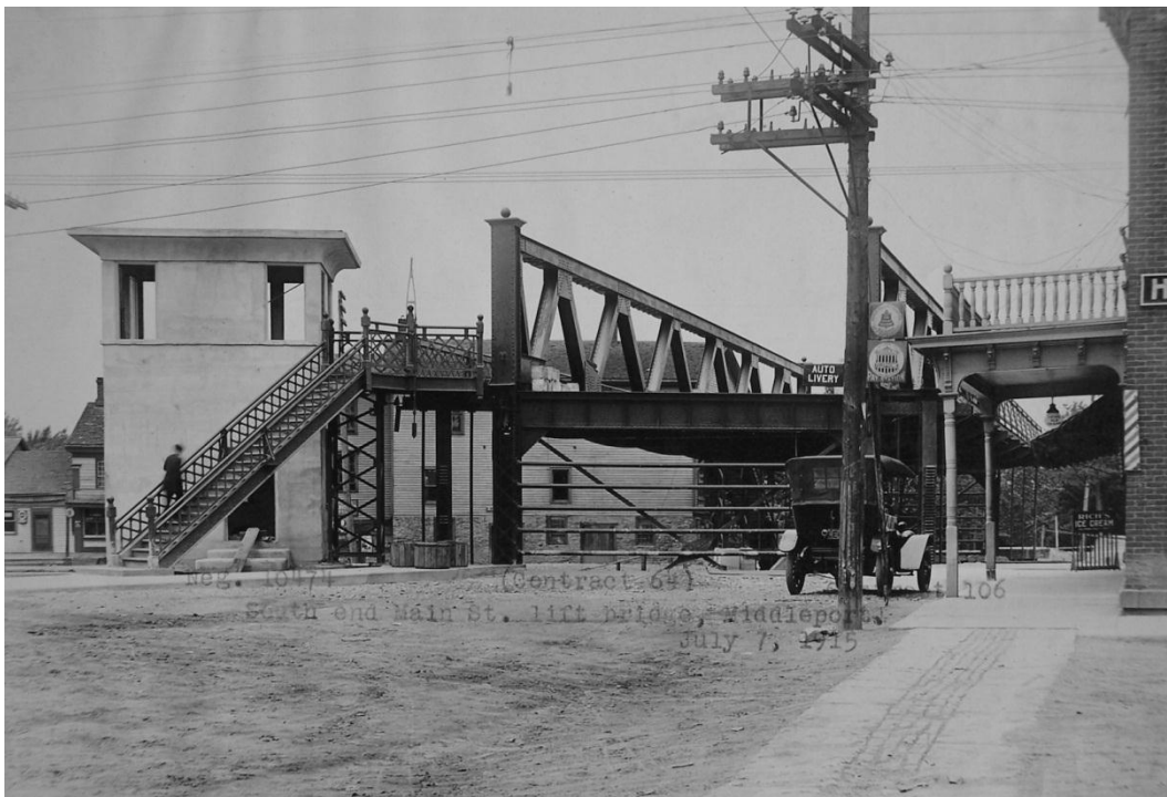
Figure 43 - Main Street lift bridge and control tower, Middleport, Niagara County, July 7, 1915 (Contract 67)
