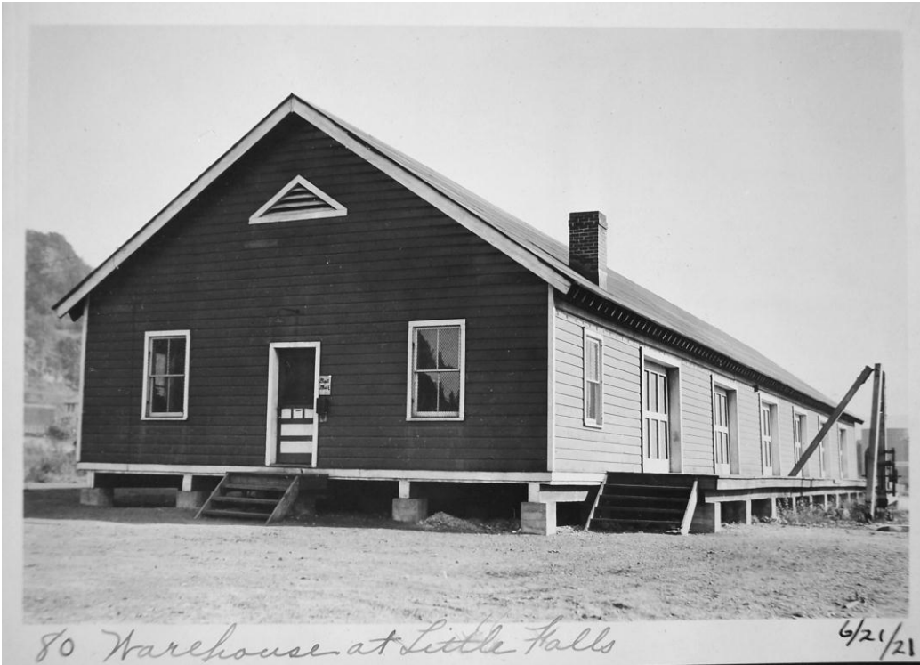
Figure 47 – Erie Canal, terminal freight house, Little Falls, Herkimer County, June 21, 1921
