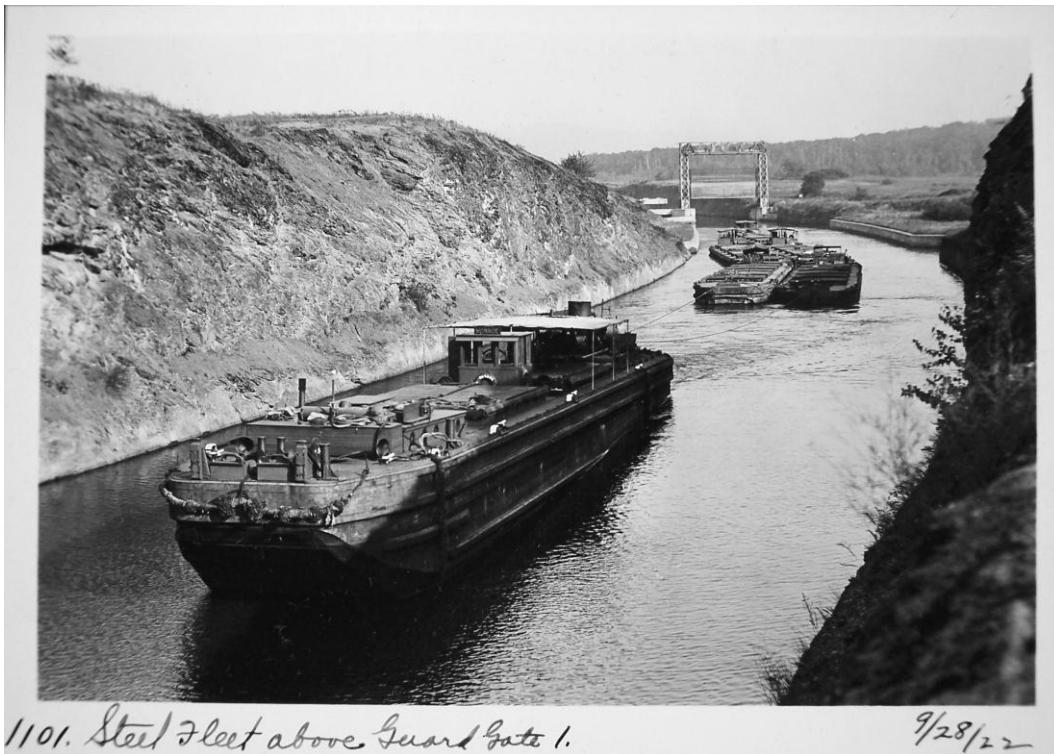
Figure 3 – Deep Cut completed, Waterford, Saratoga County, September 28, 1922
