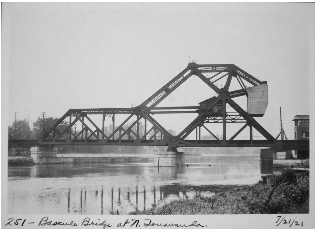
Figure 46 - Railroad bascule bridge crossing Erie Canal, North Tonawanda, Niagara County, July 21, 1921
