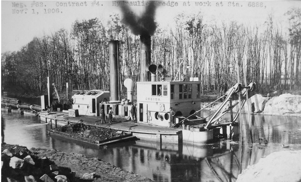
Figure 10 – Erie Canal, hydraulic dredge Oneida , east of Sylvan Beach, Oneida County, November 1, 1906 (Contract 4)
