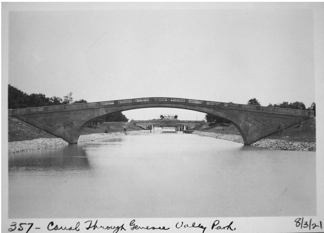
Figure 41 – Genesee Valley Park pedestrian bridges over Erie Canal, Rochester, Monroe County, August 3, 1921
