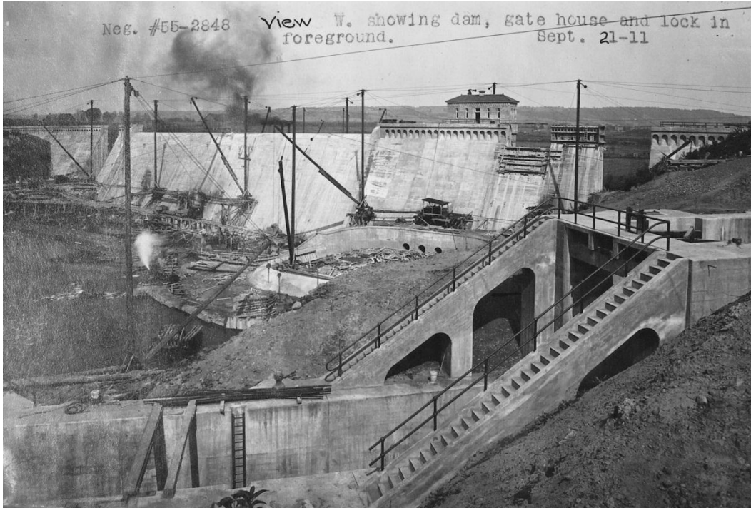
Figure 34 – Delta Dam construction, Rome, Oneida County, September 21, 1911 (Contract 55)
