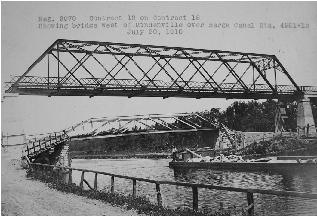
Figure 40 – Comparison of Enlarged Erie and Barge Canal bridge heights and channel widths. River Road Bridge, Mindenville, Montgomery County, July 20, 1910. (Channel Contract 18, Bridge Contract 13)
