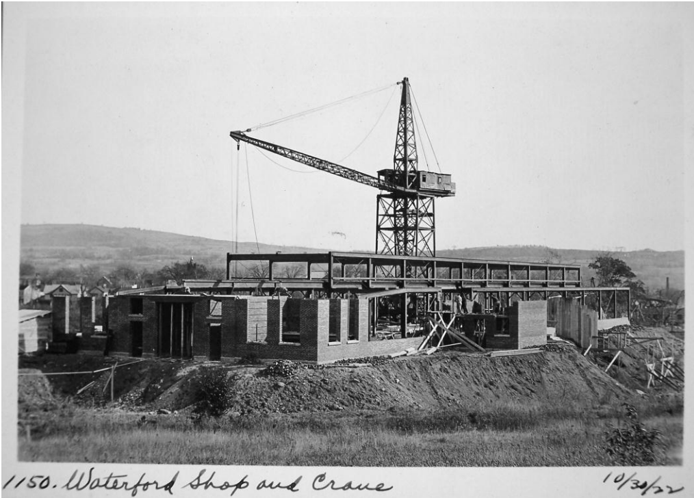
Figure 49 – Erie Canal, State Shop under construction, Waterford, Saratoga County, October 30, 1922
