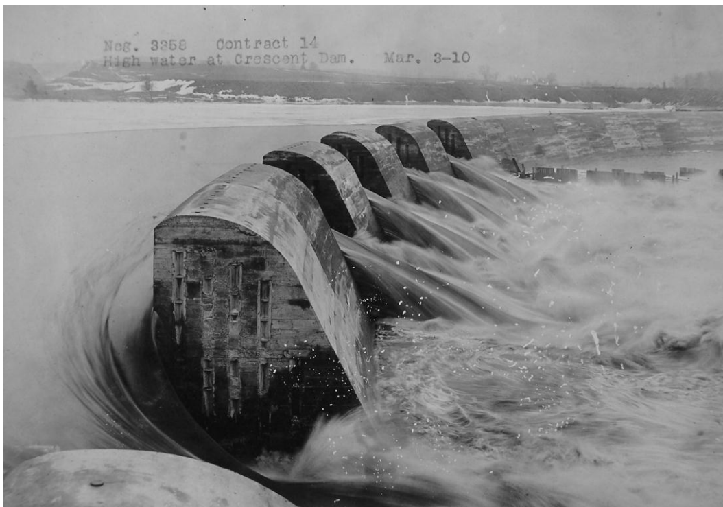
Figure 33 - Partially completed Crescent Dam during flood, March 3, 1910
