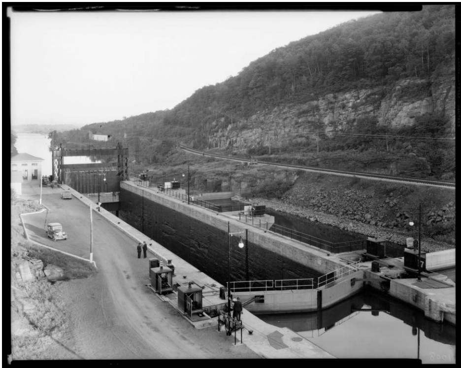
Figure 20 - Erie Canal, Lock E17, Little Falls, Herkimer County, 1930s (DPW) View from Moss Island looking southeast. Note mid-level pool in in background, built to conserve water
