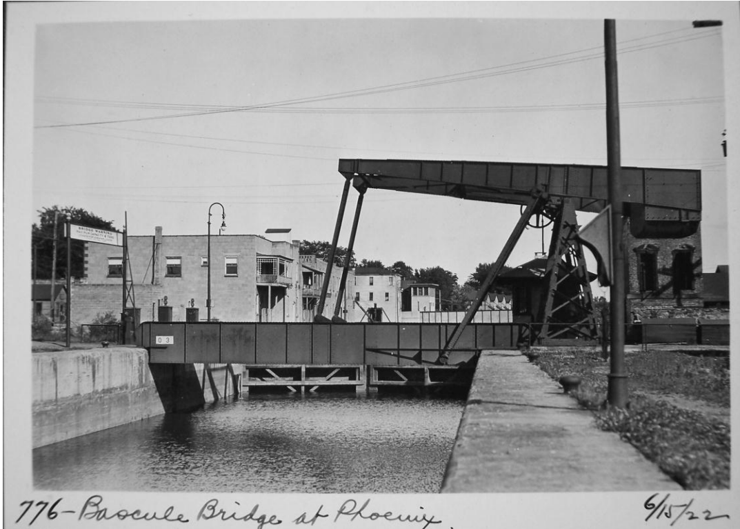
Figure 45 - Bridge Street bascule bridge crossing Oswego Canal Lock O-1, Phoenix, Oswego County, June 15, 1922
