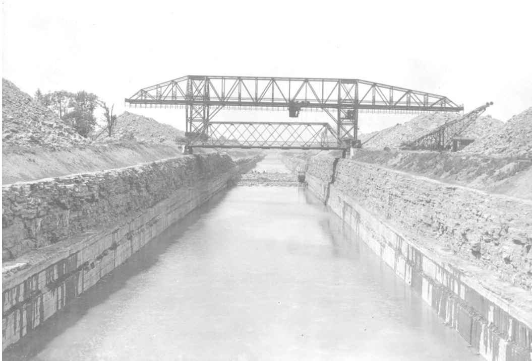
Figure 4 - Erie Canal, "Grab Machine" Deep Cut, Rochester, Monroe County, ca. 1909 (Contract 6)
