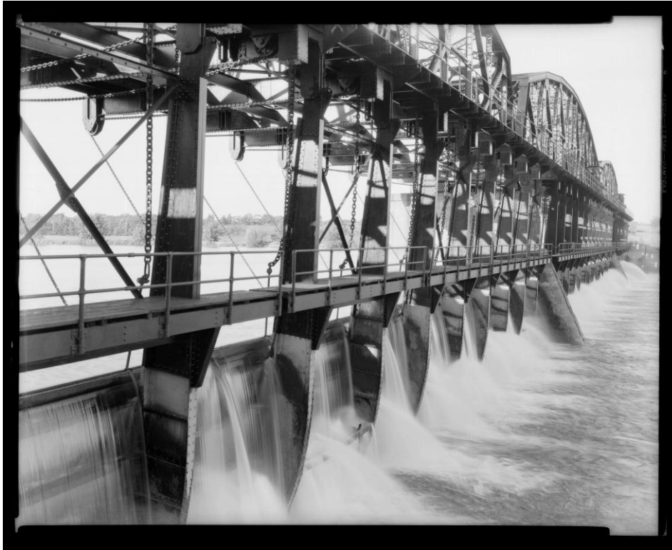
Figure 17 – Erie Canal, movable dam at Lock E8, Rotterdam, Schenectady County, 1930s (DPW)
