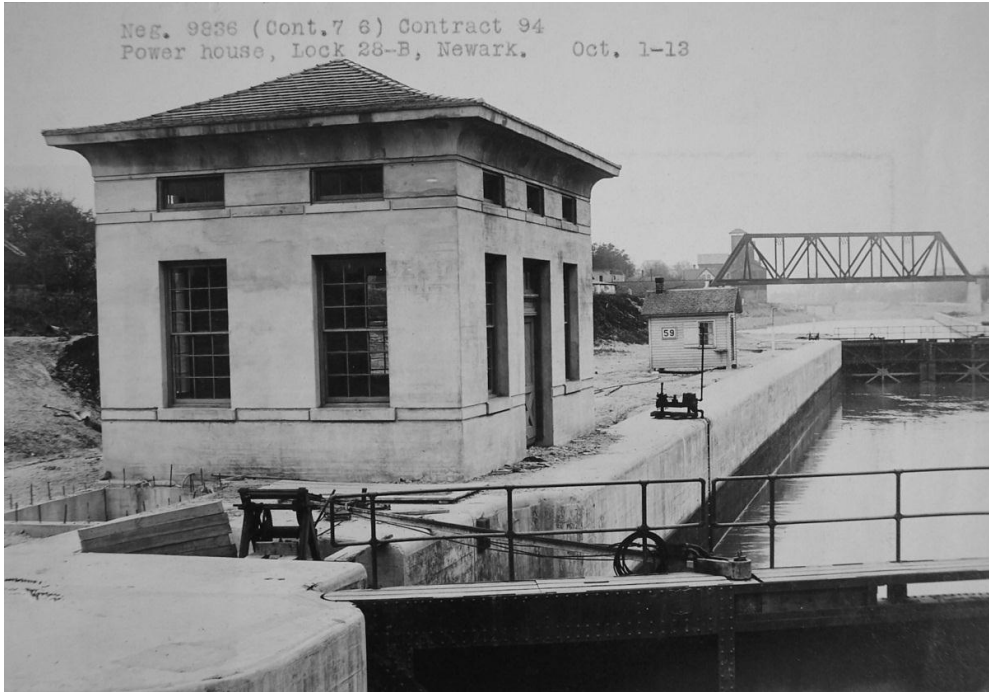
Figure 28 – Erie Canal, Powerhouse, Lock E28B, Newark, Wayne County, October 1, 1913 (Contracts 76 & 94) Note reuse of old shanty from nearby Enlarged Erie lock 59
