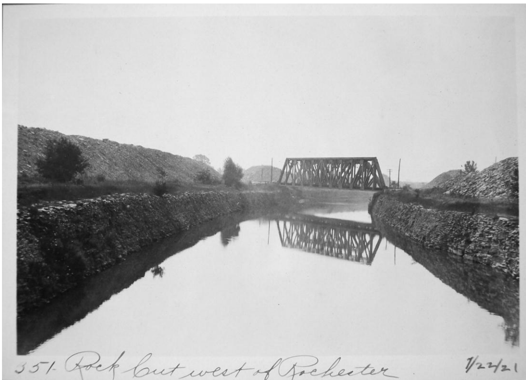
Figure 5 - Deep Cut completed, Rochester, Monroe County, July 22, 1921
