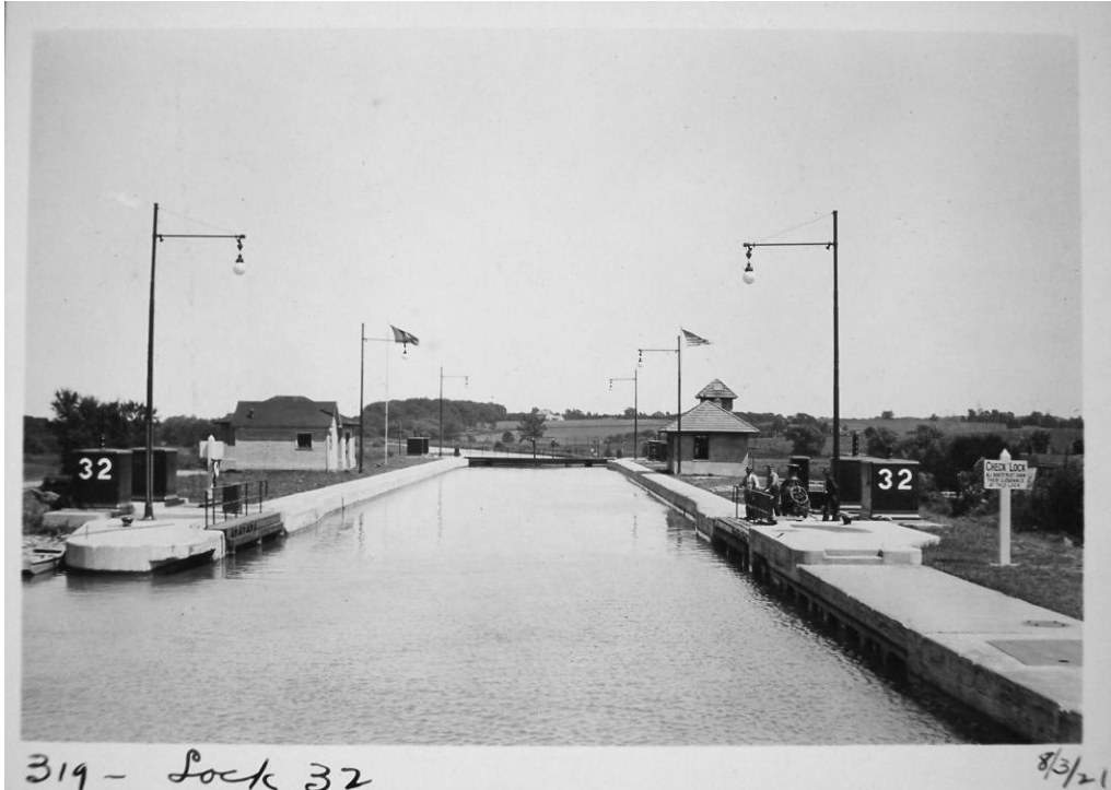
Figure 23 – Erie Canal, Lock E32, Pittsford, Monroe County, August 3, 1921
