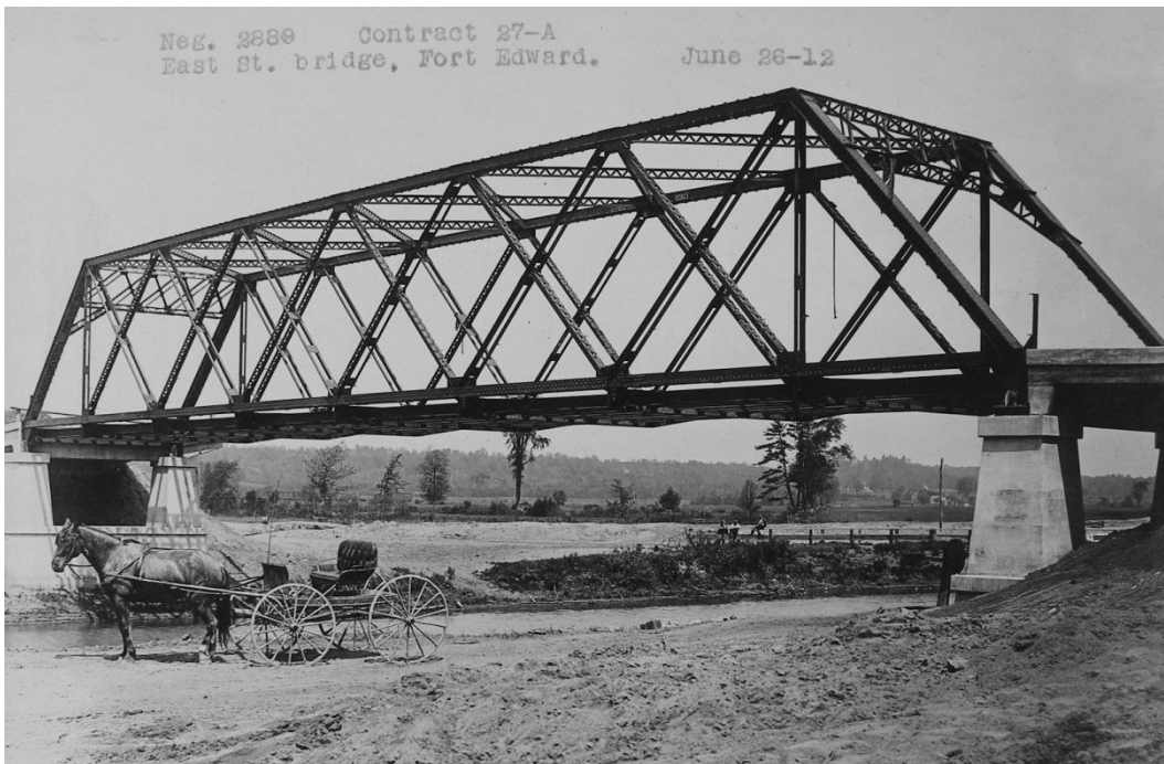
Figure 39 - East Street Bridge over Champlain Canal, Fort Edward, Washington County, June 26, 1912 (Contract 27-A) Double-intersection Warren trusses were erected at many locations across the Barge Canal. The configuration is not common outside New York.
