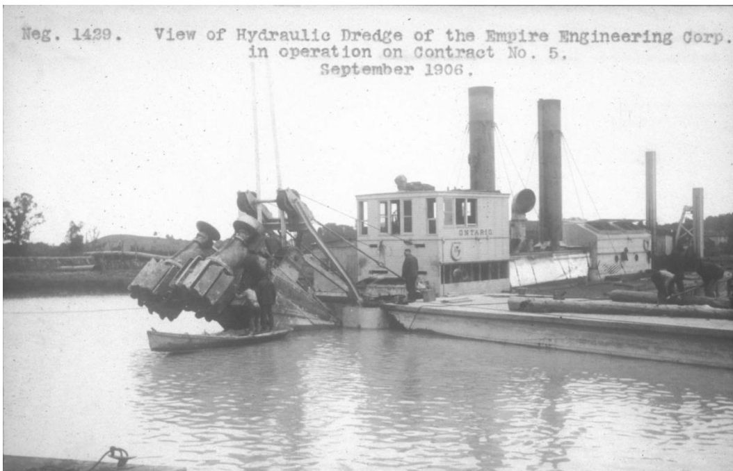
Figure 9 – Erie Canal, Hydraulic Dredge Ontario with cutters raised, near Montezuma, Cayuga County, September 1906 (Contract 5)
