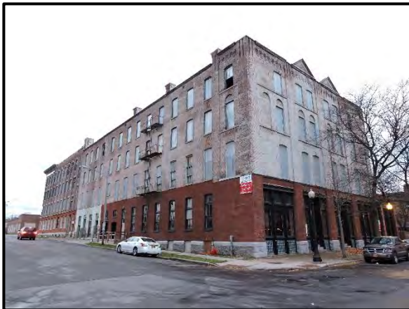
Doyle Hardware Building (Main Street façade).
