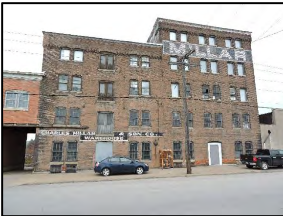
Buildings A and B.
