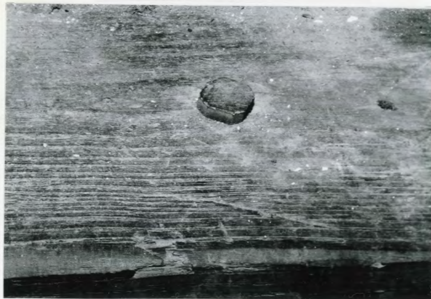
#19- Pegged cellar step
