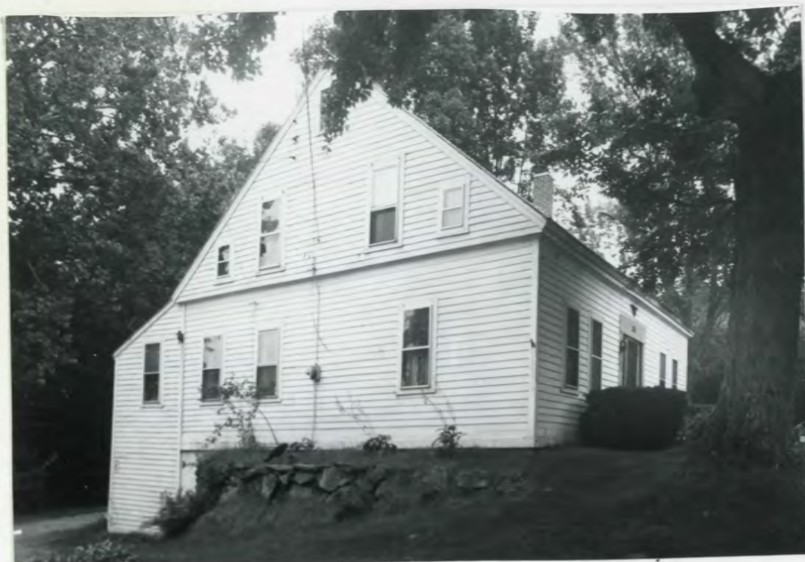
#3- N end & W front elevations
