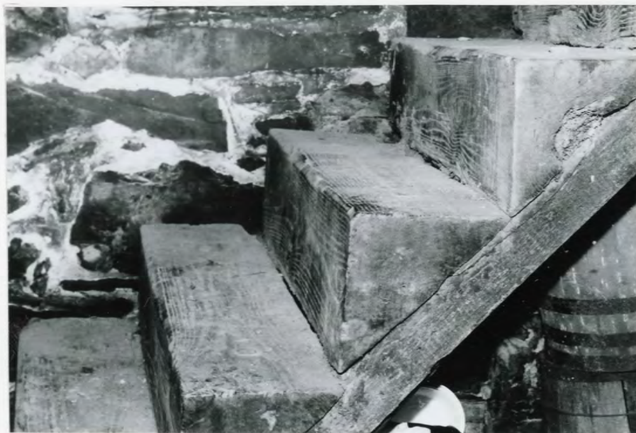
#18- Cellar steps from diagonally sawed timber
