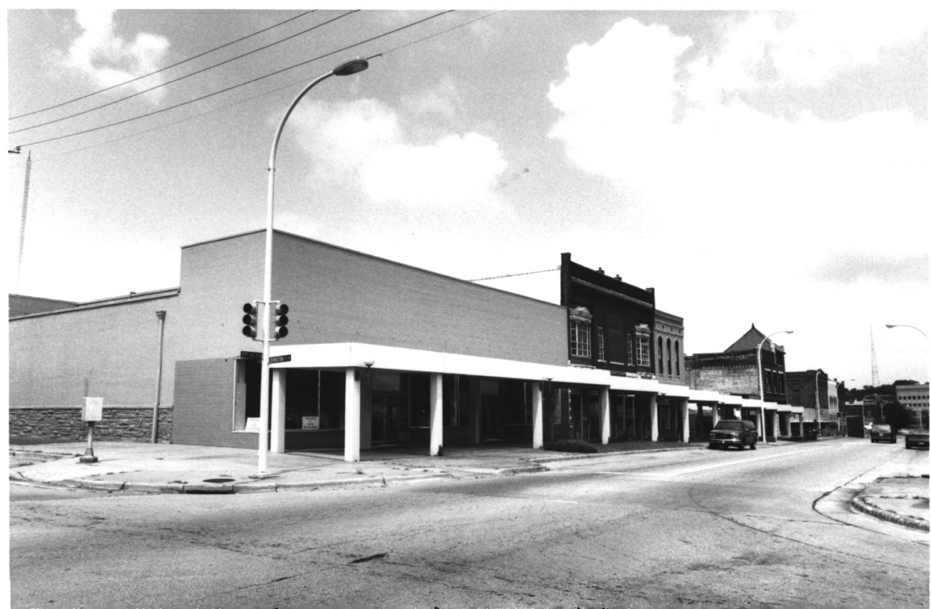
Photo # 11: Streetscape, 100 Block 2nd Ave. S.E. Decatur, Albany, Herndon Commercial Hist. Dist. Morgan Co. AL
