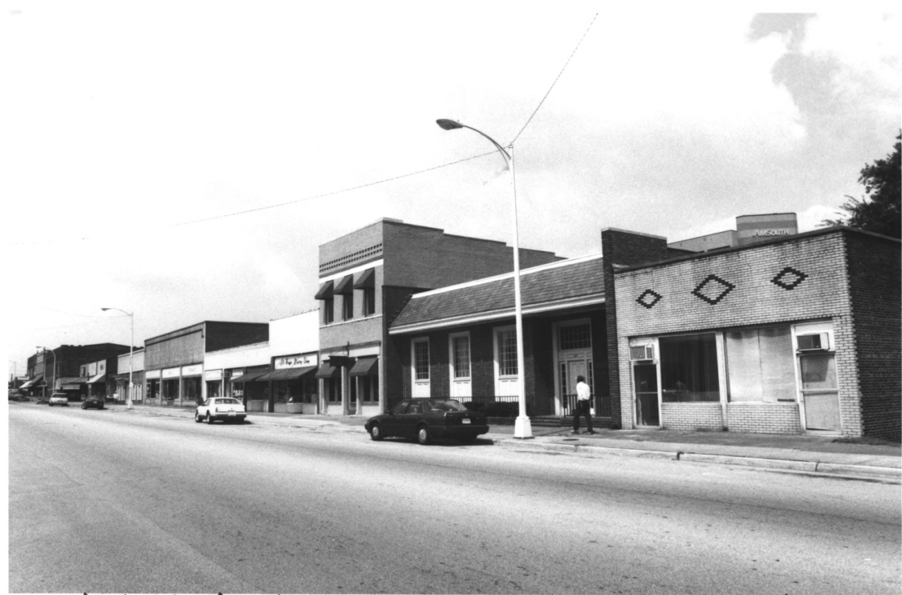
Photo #8: Streetscape, 200 block E. Moulton St. Decatur, Albany Meridian Commercial Blvd. Dist. Morgan Co. AL
