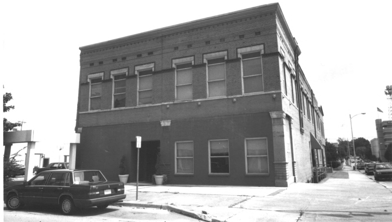
Photo #116: 224 2nd Ave. S.E. Albany Heritage Commercial Dist. Dist. Morgan Co. AL Decatur, Morgan Co. AL
