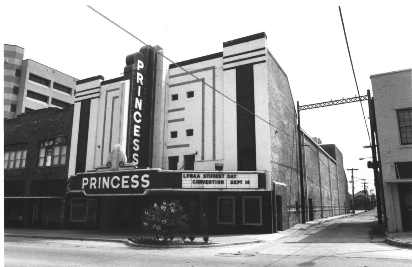
Photo #3: 112 2nd Ave. N.E. Albany Heritage Commercial Bldg. Dist. Decatur, Morgan Co.
