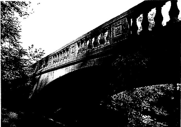
View Looking Up at the South Side of the Bridge.
