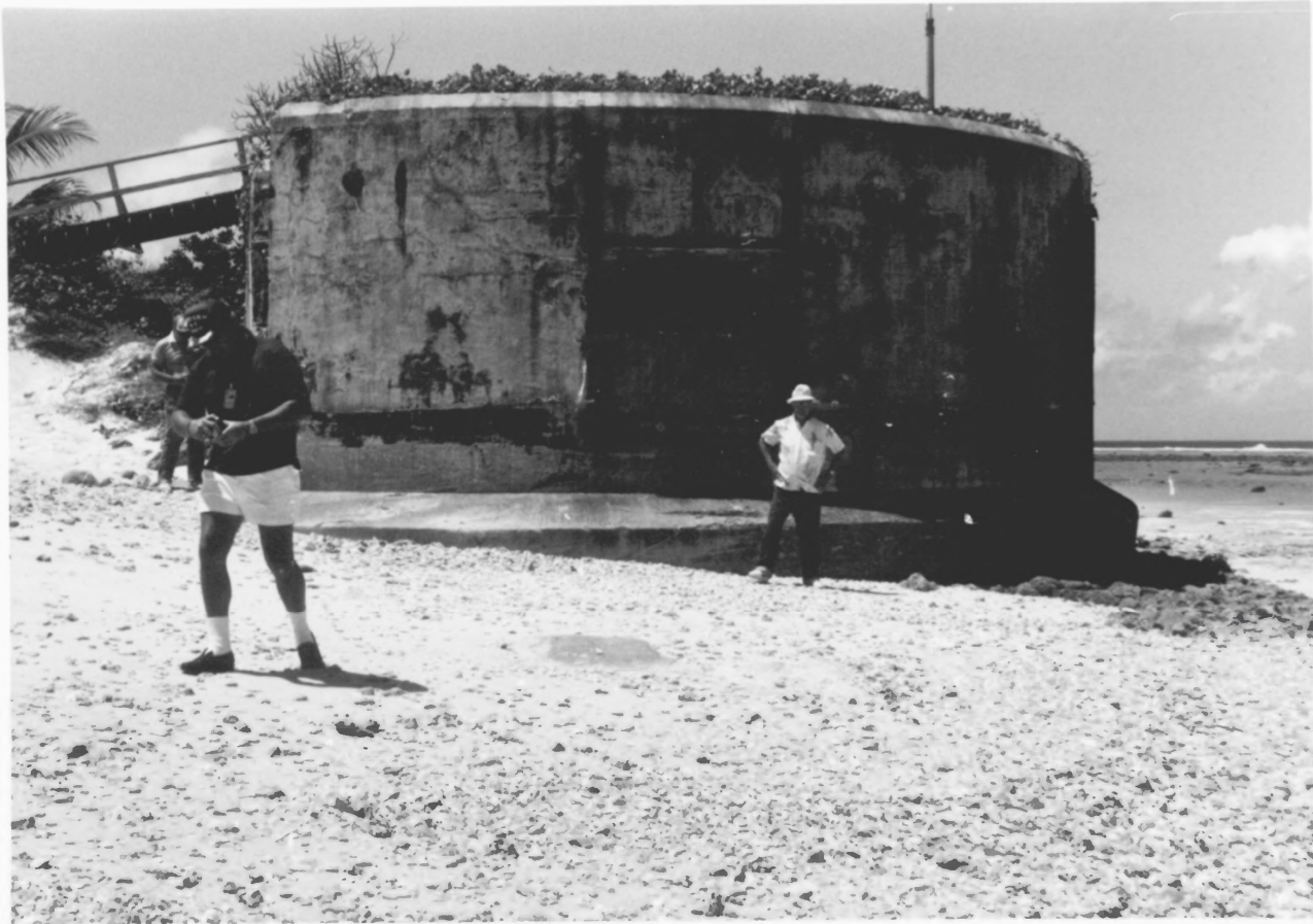
6. Japanese circular blockhouse on Roi. There were four or five (accounts differ) of these strong defensive works on Roi-Namur. American intelligence personnel thought they were of German design. This one, at the northwest corner of Roi, is the best preserved of three survivors. The person with the white shirt is standing in front of one of four gun embrasures.
