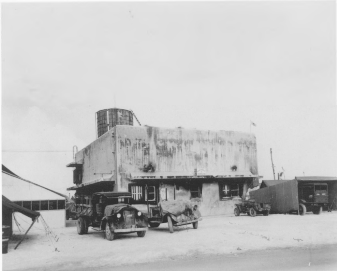
10. Japanese power house on Namur. Here, the Fourth Marine Air Wing is using it as a dispensary, June 26, 1944. Kwajalein Missile Range still makes use of the structure. In the foreground are two Japanese trucks that Marines put to good use.
