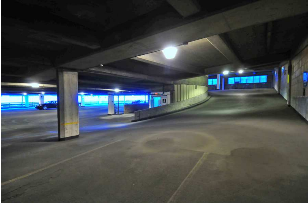
Figure 20: Commerce Garage, fourth floor, view southwest. Source: Brad Finch, F-Stop Photography, October 2014.
