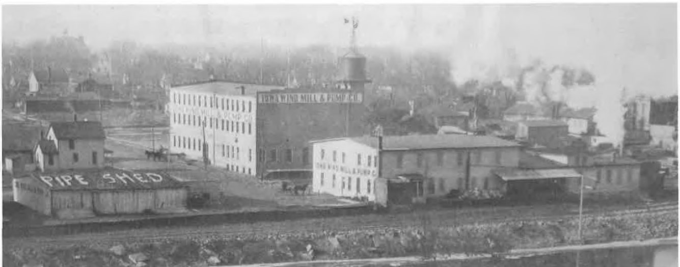
Top: 1904 advertisement with photographs of plant at its peak looking West; also company executives. Bottom: Close-up detail of c. 1904 photograph. Source: Cedar Rapids Evening Gazette , January 9, 1904. Copy provided by the Carl and Mary Koehler History Center, Archives, Cedar Rapids, Iowa.
