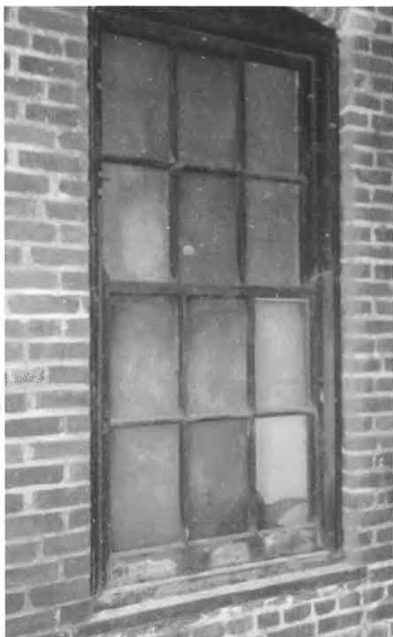
Original window on 2nd floor NW corner interior
