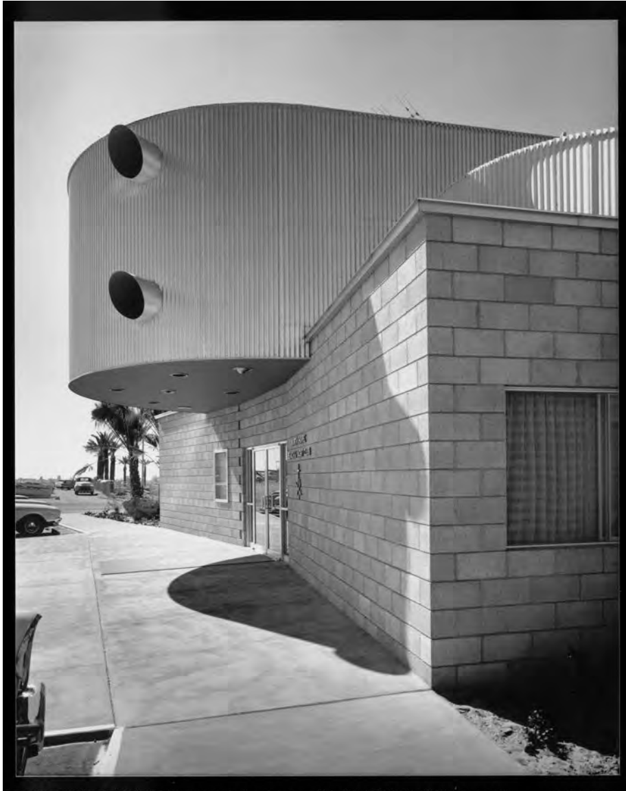
Figure 3. Northeast elevation, looking south, 1960.
