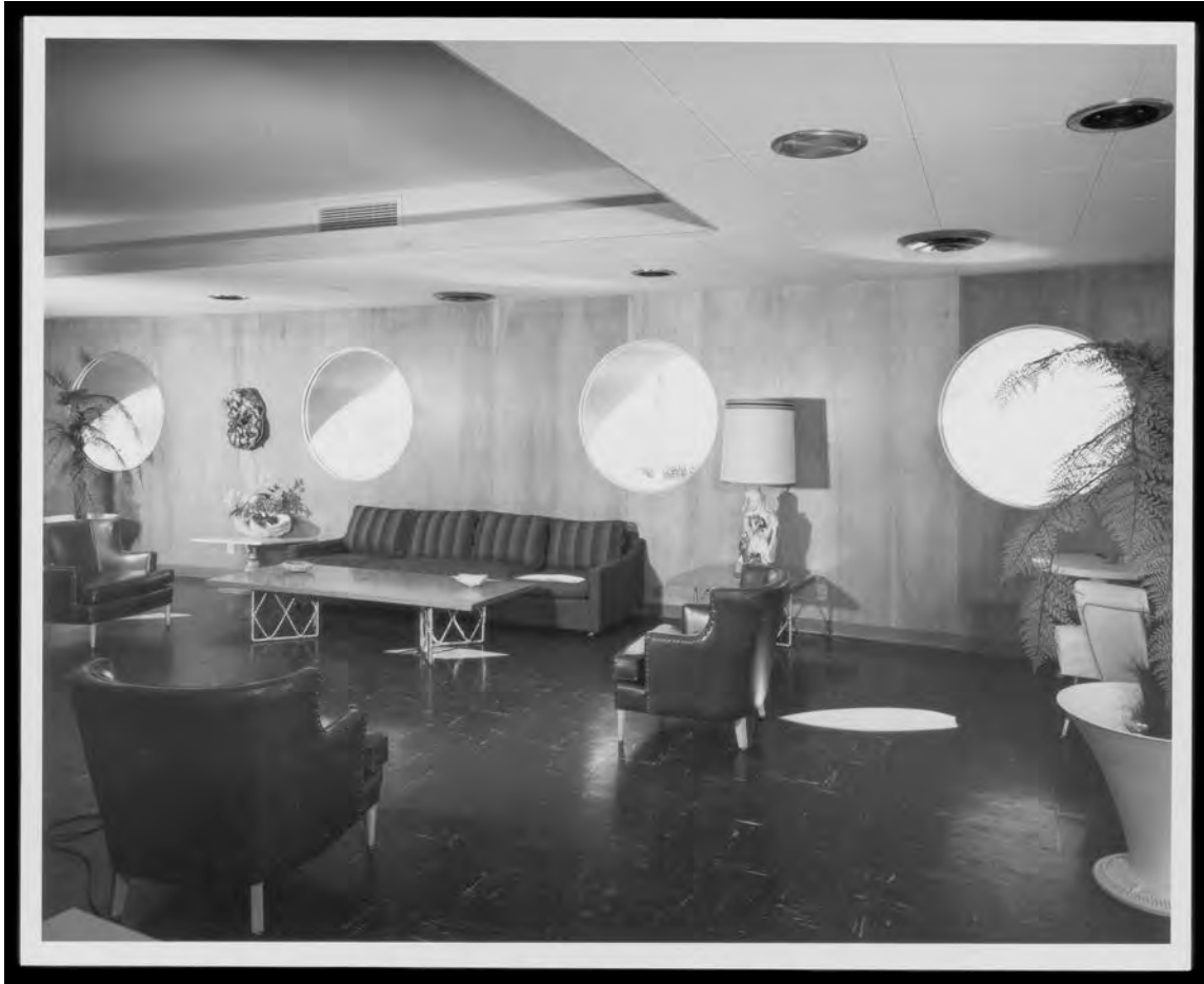
Figure 4. Interior view, second story, looking southwest, 1960.
