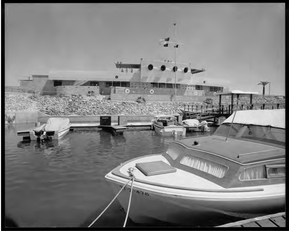
Figure 2. Southwest elevation, looking east, 1960.
