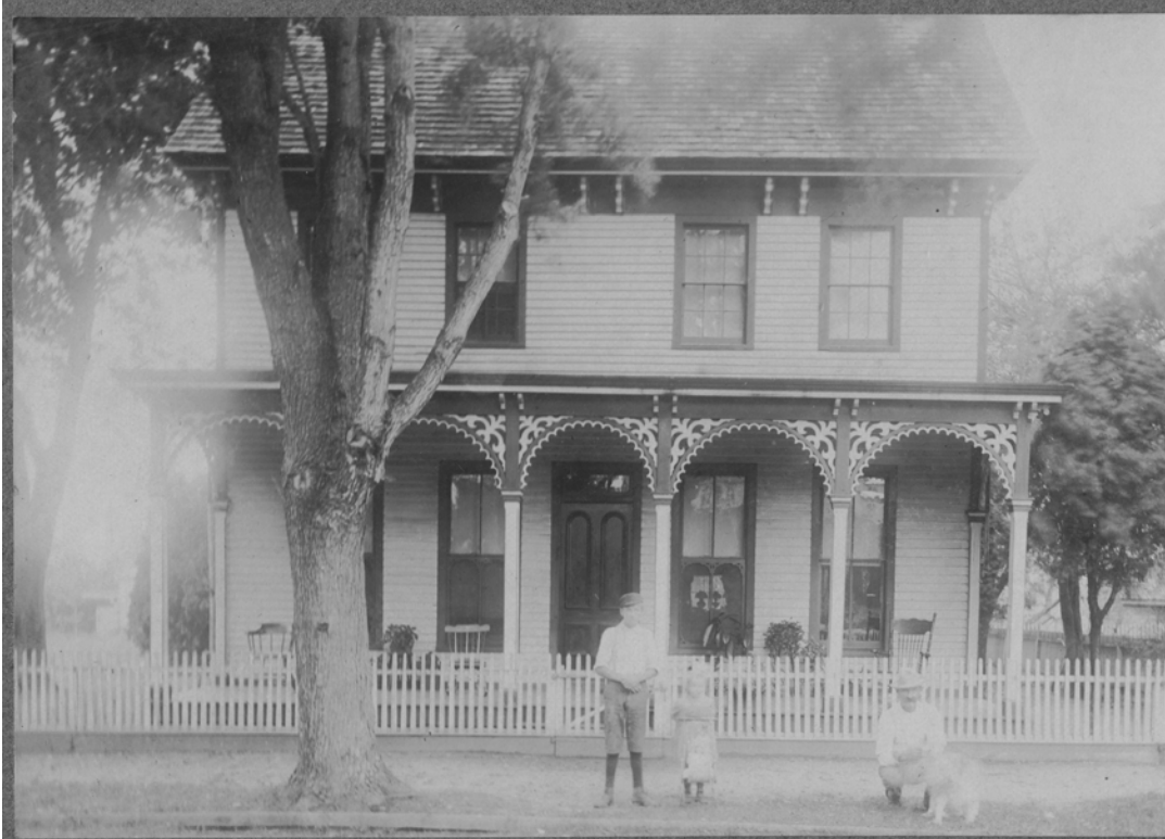
Historic Photo 13.: Historical view of 9536 Highland Street (extant). The building is identified as the “D. Wills” house on the 1876 Atlas Map.
