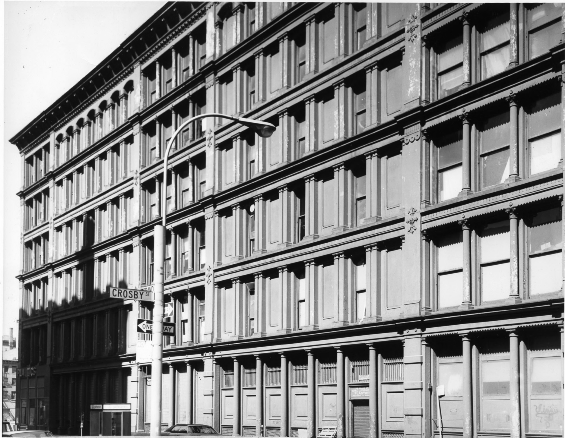
SoHo-Cast Iron Historic District, N.Y.
