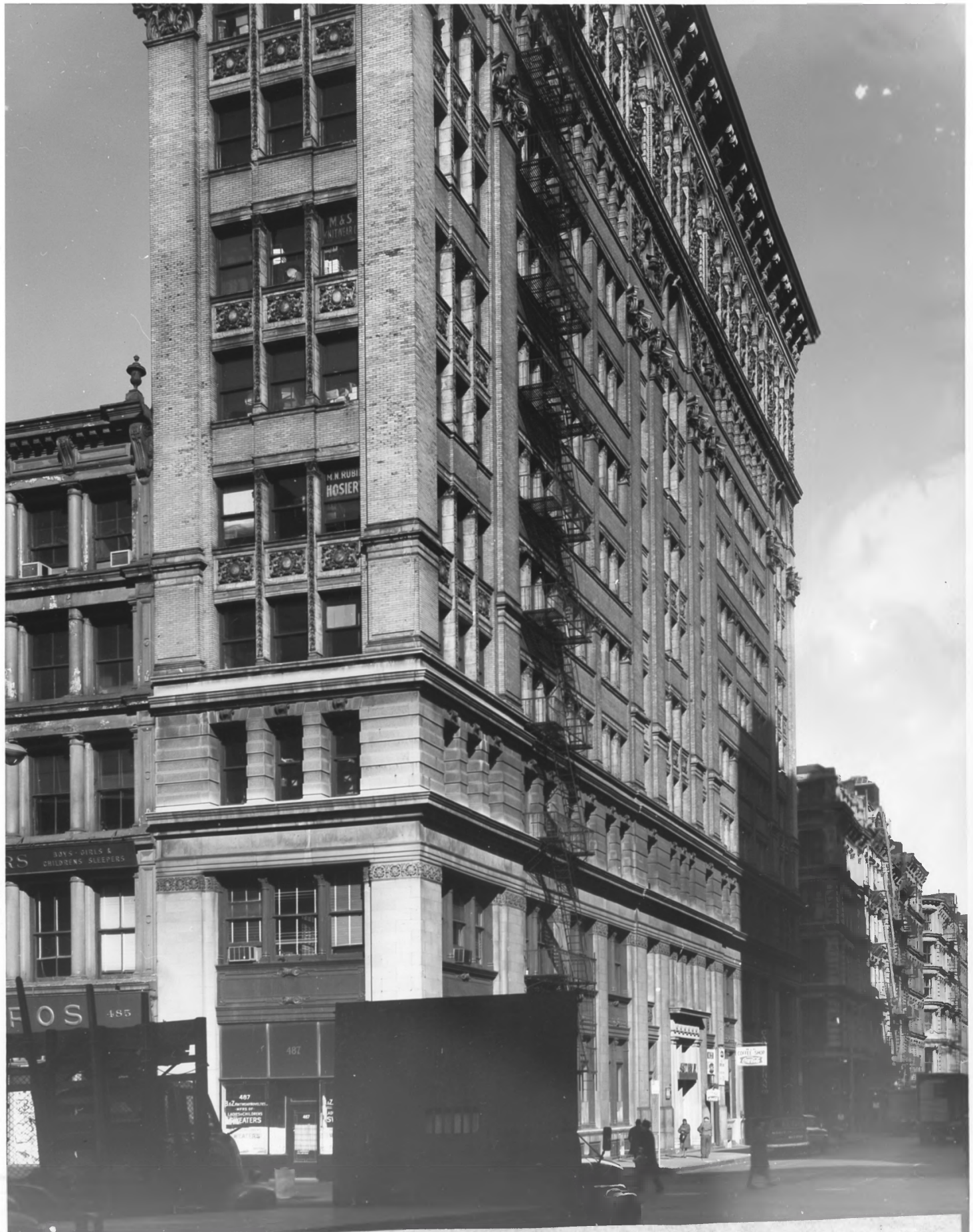
SoHo-Cast Iron Historic District, N.Y.
