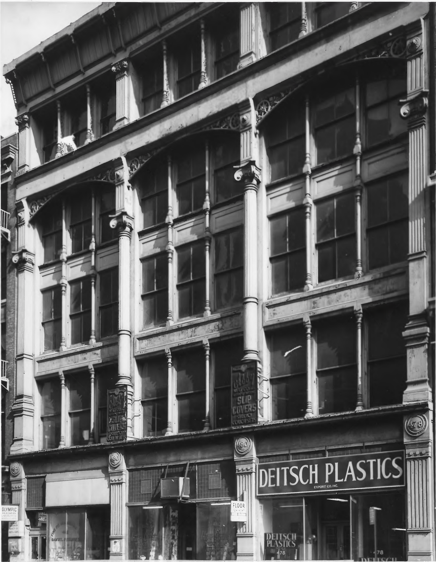
SoHo-Cast Iron Historic District, N.Y.
