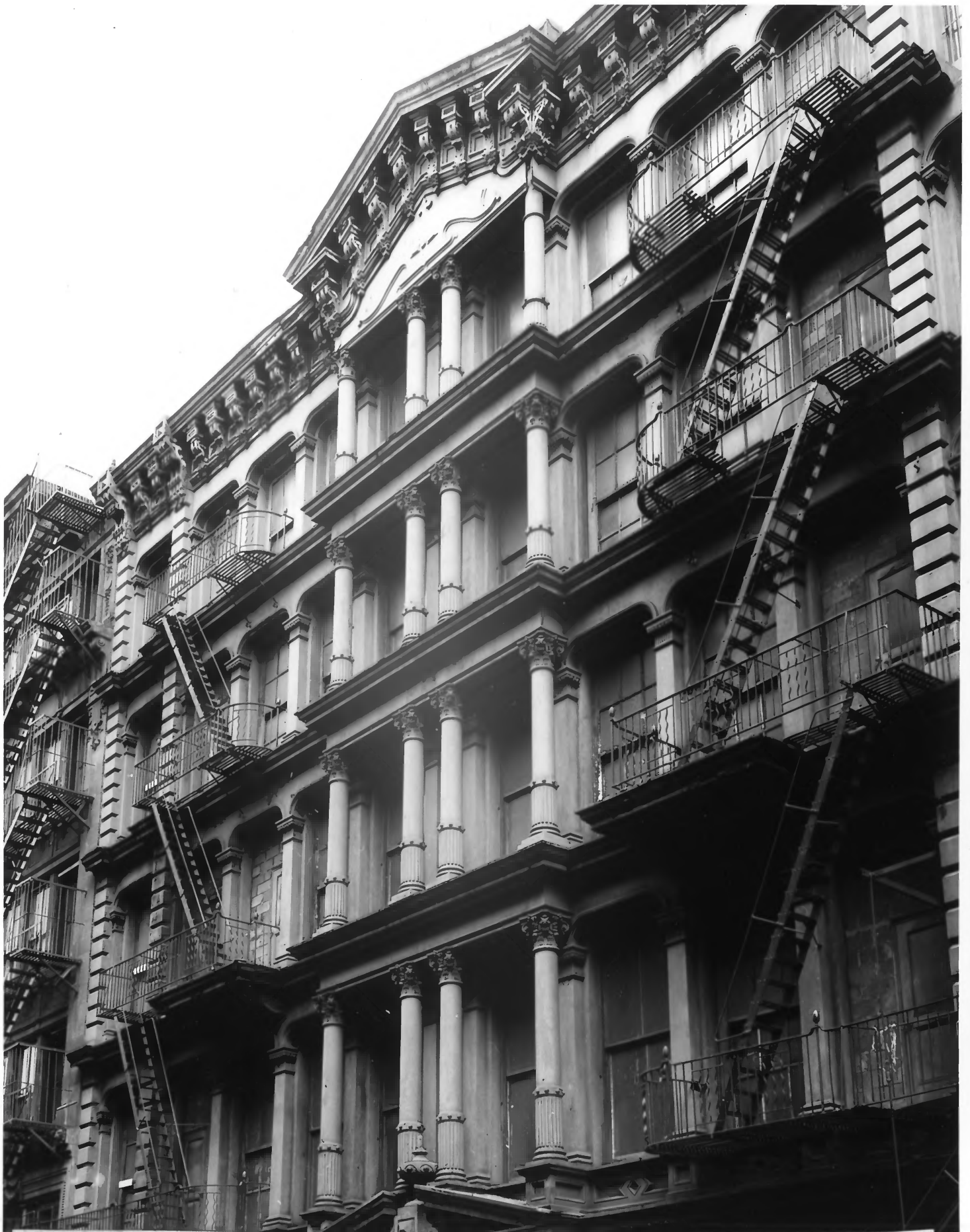
SoHo-Cast Iron Historic District, N.Y.
