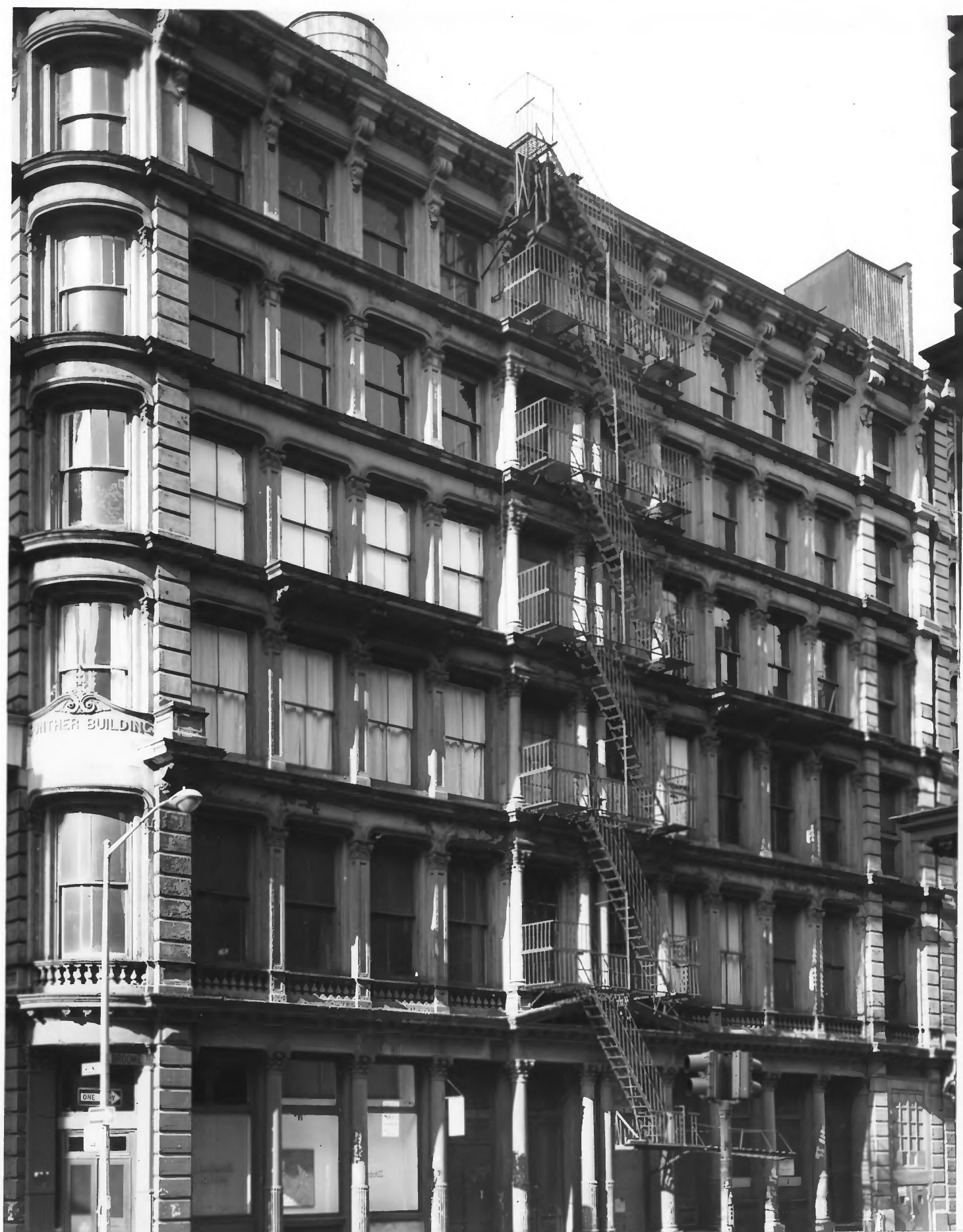
SoHo-Cast Iron Historic District, N.Y.
