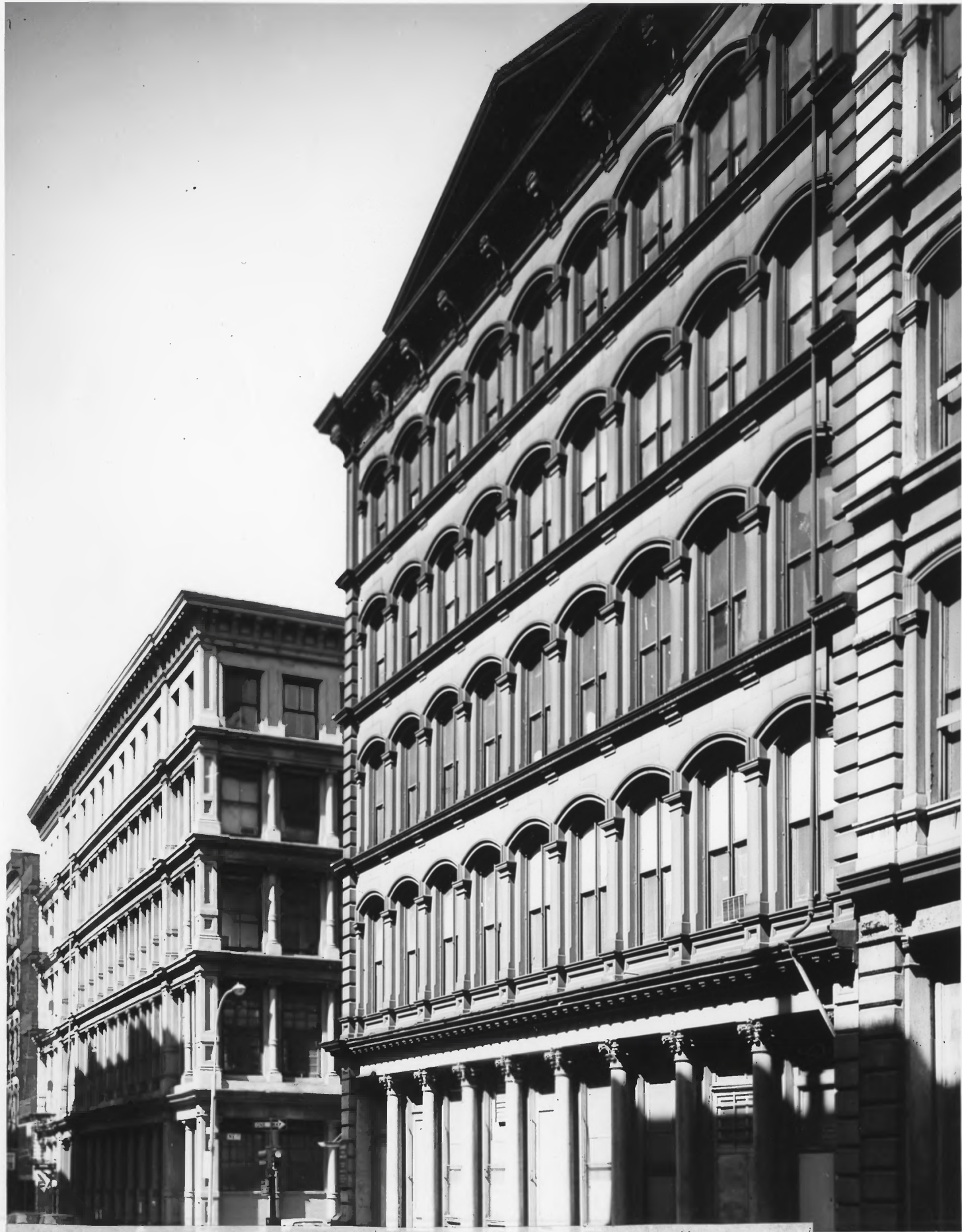
SoHo-Cast Iron Historic District, N.Y.
