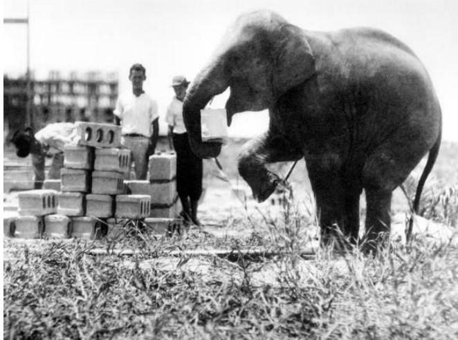
Figure 5: 1923 photograph of Rosie the Elephant moving concrete blocks at the construction site of the Nautilus Hotel. Carl Fisher purchased two elephants to serve as the mascots of Miami Beach in promotional images. Rosie was an extremely popular figure in early Miami Beach, performing at public events, including serving as United States President-elect Warren G. Harding’s golf caddy when he visited the city in 1921. Source: Florida Memory
