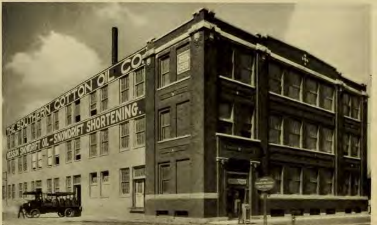
Southern Cotton Oil Building, 37th Street and Laffin Place. This concern is one of the largest dealers in cotton oil products, paints and similar lines, in the country. Formerly located at 32nd Street, on the Burlington Road. Building brick and fireproof construction, containing about 73,000 square feet of floor space, erected in 1910. A. S. Alschuler, Architect; Joseph Haigh & Sons Co., General Contractors. An additional cooperage shop was erected in 1914, which has about 10,000 square feet of floor area. This is also of concrete construction. Architect, S. Scott Joy, District Architect; E. W. Sproul Company, General Contractor.
