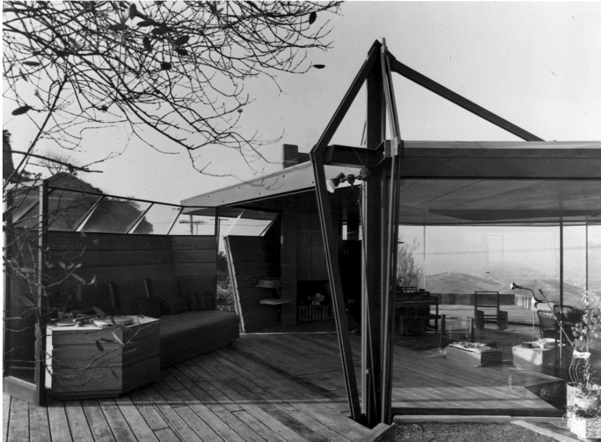
View of pivoting wall and roof support on south façade, facing northwest (© The John Lautner Foundation, courtesy of Frank Escher, date of photograph unknown)
