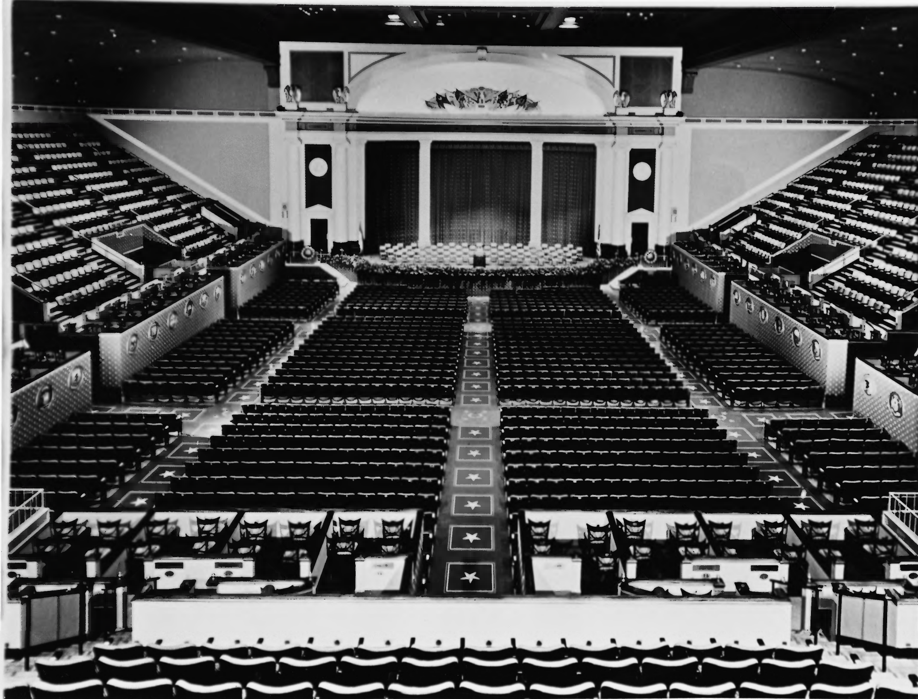
The Auditorium, Constitution Hall. The hall has been praised for its excellent acoustics. Note the absence of pillars that would obstruct the view of the audience. (Courtesy NSDAR, 1985)
