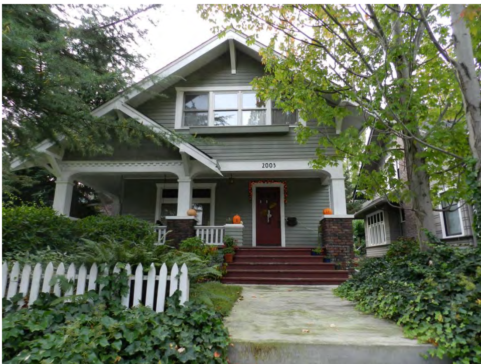
32 of 38 2003 25th Ave. E. Primary façade looking west
