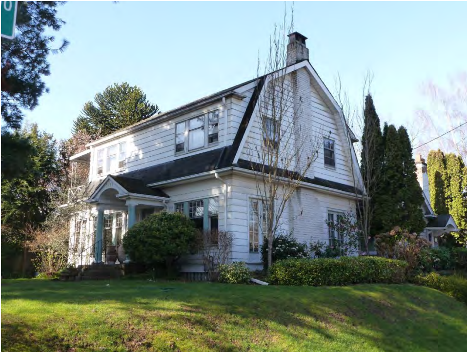
29 of 38 2111 22nd Ave. E. Gilbertson Residence Primary façade looking northwest Connie Gray 3/4/2015
