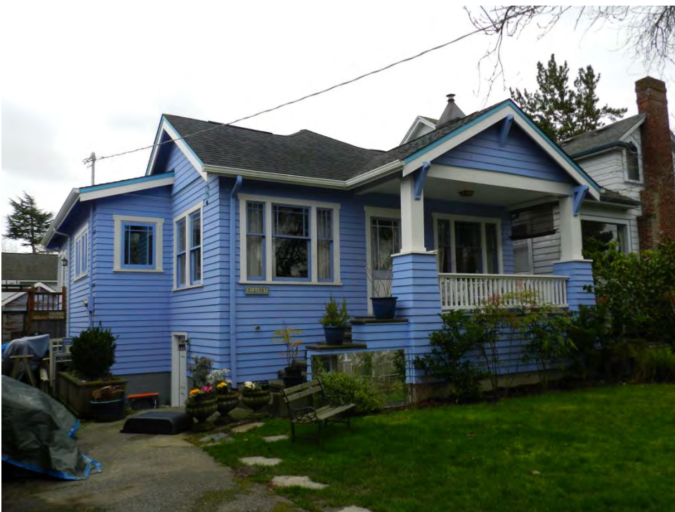
24 of 38 2507 E. McGraw St. Skinner Residence Primary façade looking south Connie Gray 2/27/2014
