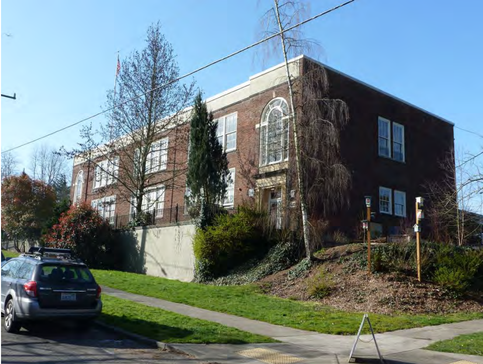
19 of 38 2405 22nd. Ave. E. Montlake School northeast corner/entry looking southwest Connie Gray 3/4/2015
