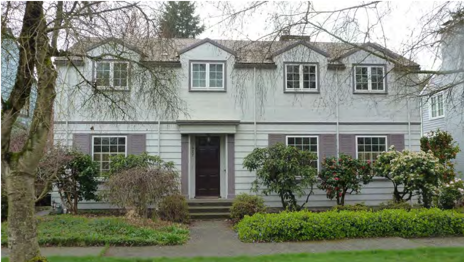
17 of 38 1627 E. Calhoun Knudson Residence Primary façade looking south Connie Gray 3/26/2014
