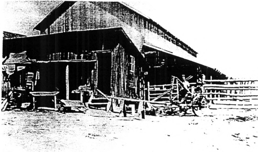
Figure 3. Blacksmith Shop and Cow Barn. The Blacksmith Shop (Resource Number 14), foreground, and Cow Barn (Resource Number 15) appear in this undated, circa 1900-1910 photograph. SOURCE: Quentin Baker, Longmont, Colorado.
