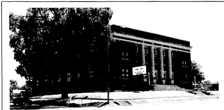
Independence Memorial Hall Southeast corner Pennsylvania Avenue and East Locust Street
